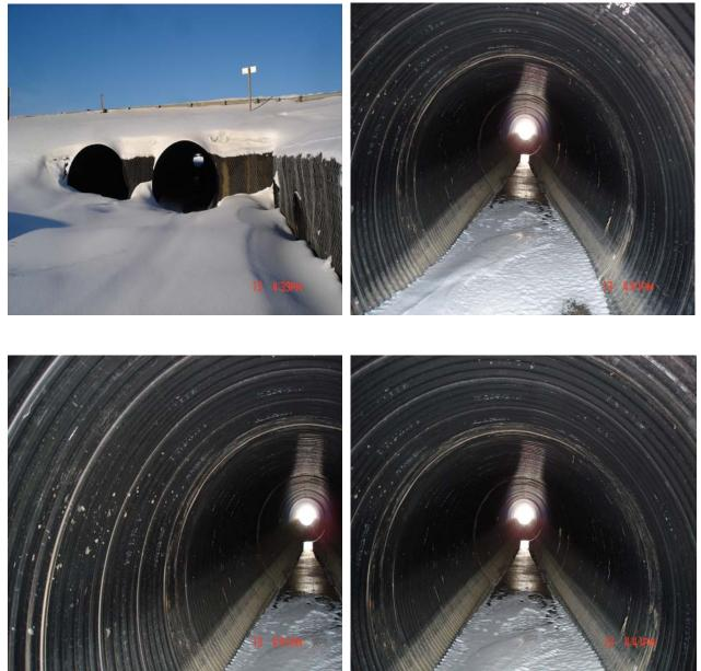
Polymer coated CSP's are performing well, with no signs of coating problems visible. Need to access yearly. Product is currently under the Trial category of AIT's products list.
