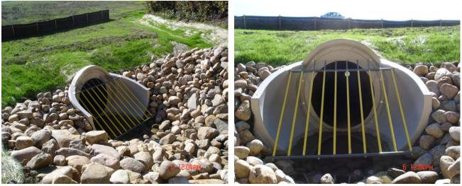
Upstream end, End treatment with grate (1200 mm dia.)
