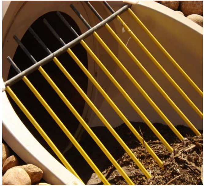
Upstream end, End treatment with grate (1200 mm dia.)
