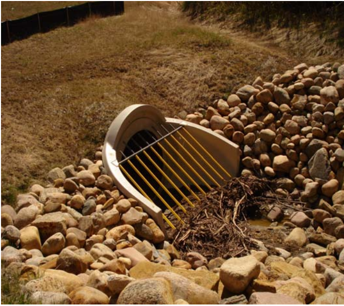
Upstream end, End treatment with grate (1200 mm dia.)
