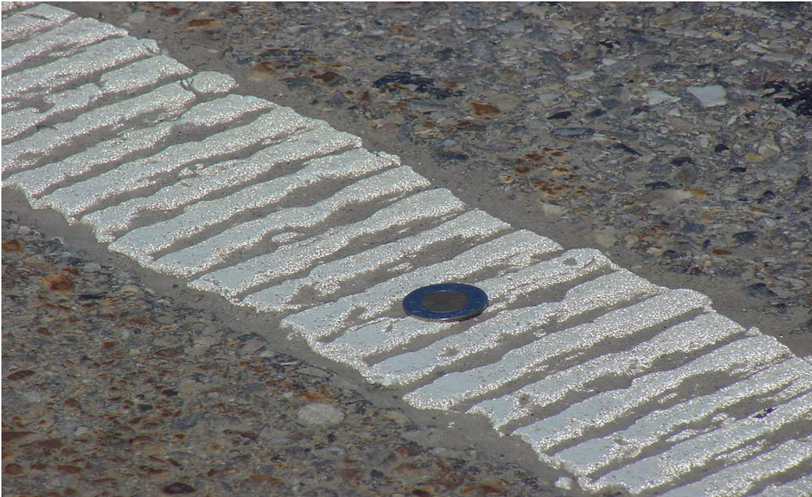
Close up look at the Rainline marker notice the excellent glass bead retention.
