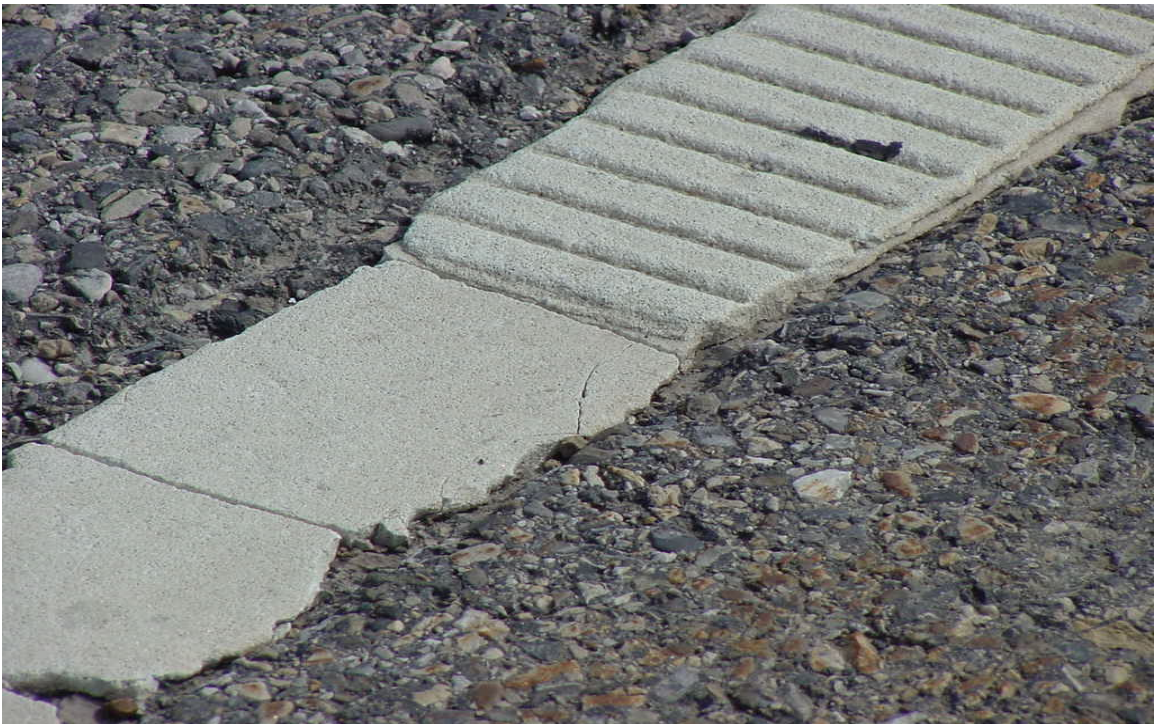
There is a section of Rainline that transitions to a thin layer of thermoplastic without the grooves. I assume this was done to compare the performance of each one.
