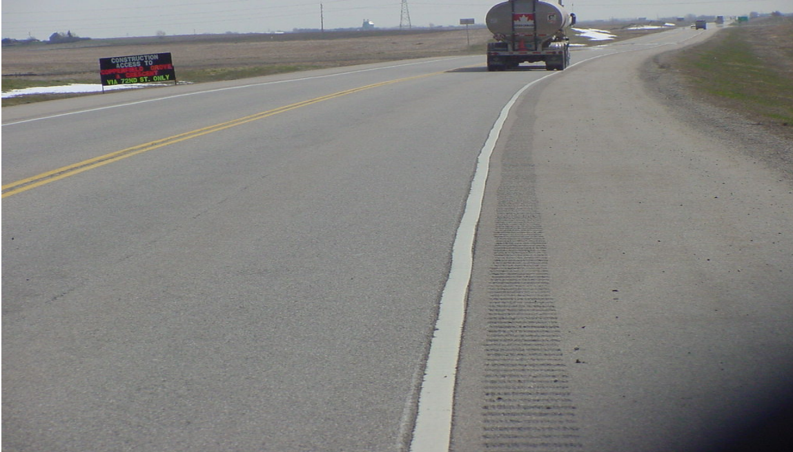
Rainline right edge line providing very good delineation.
