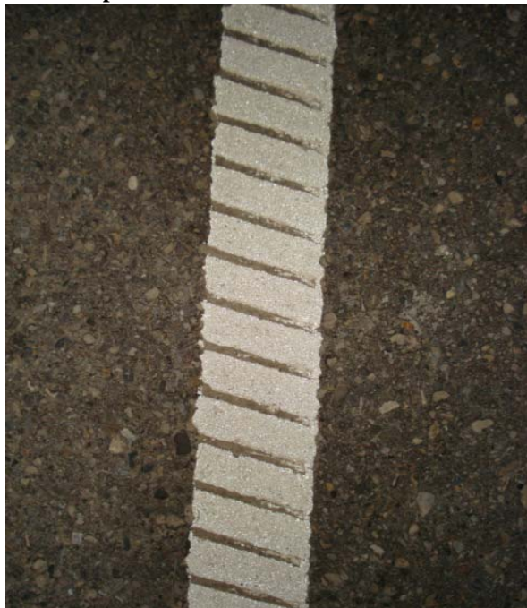
White skip line showing some chipping. Very good glass bead retention.
