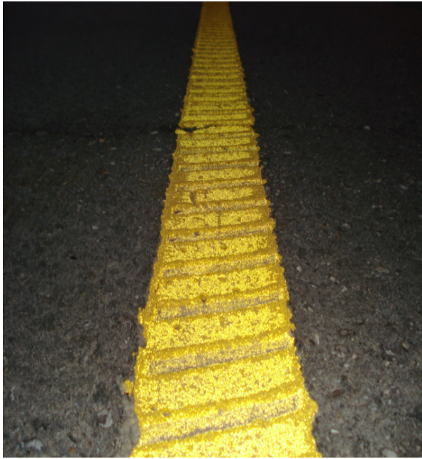
Yellow edge line looks very good with excellent glass bead retention
