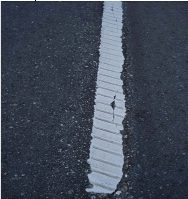
Some failure on skip lines
