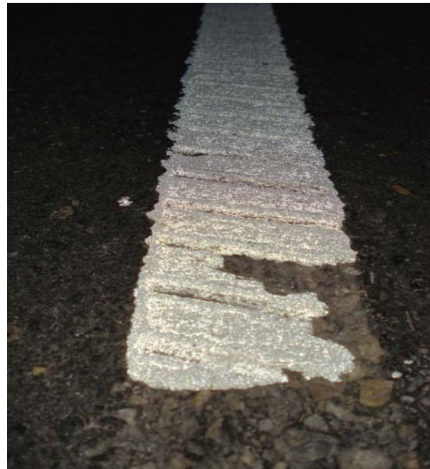
Some failure on skip lines
