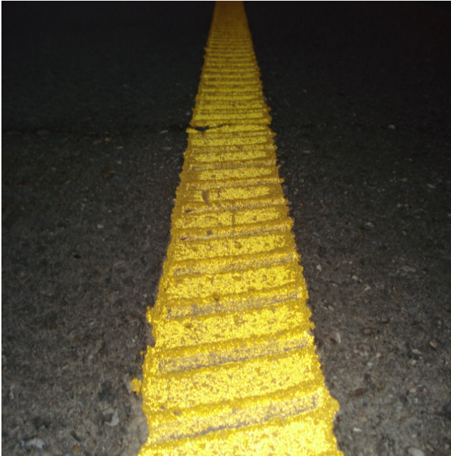
Yellow line looks in good shape with good glass bead retention.
