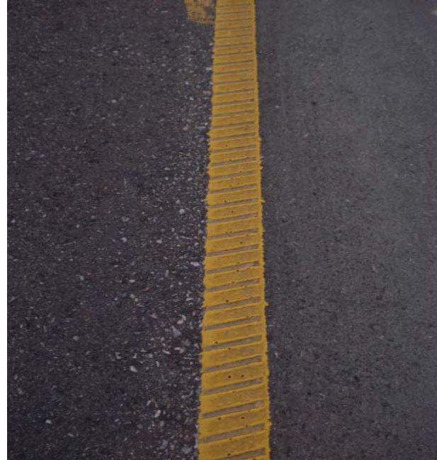
Yellow line looks in good shape with good glass bead retention.
