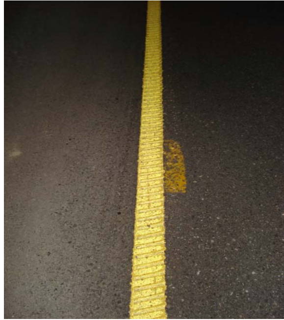
Yellow edge line looks very good with excellent glass bead retention
