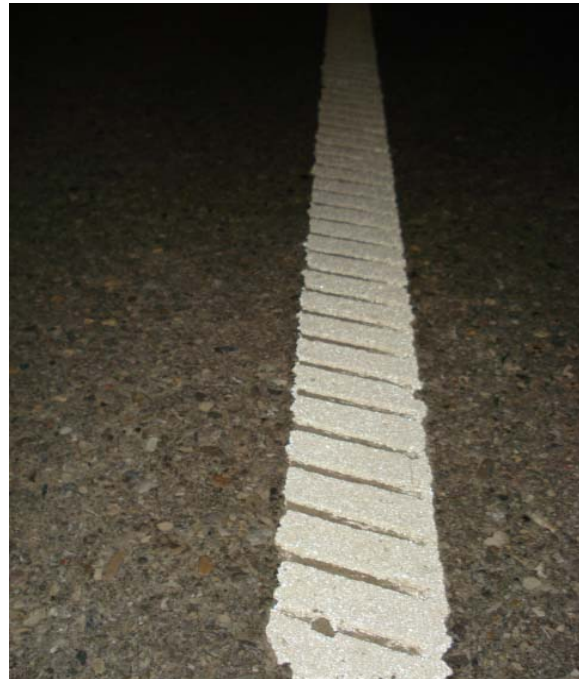
White skip line showing some chipping. Very good glass bead retention.
