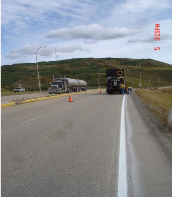
Application of Rainline
