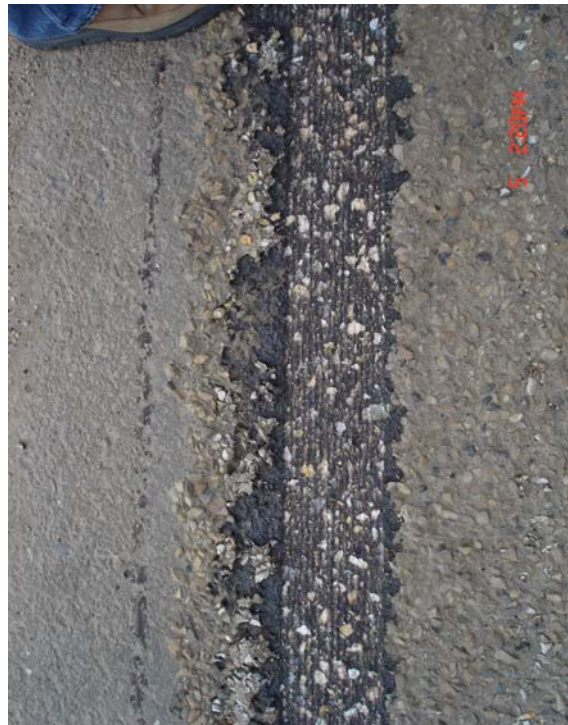
Double seal coat on bridge, edge failure
