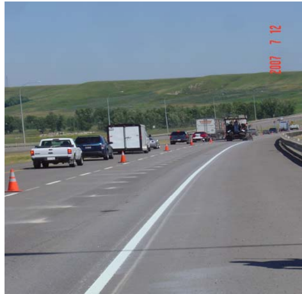
Fresh Rainline marking
