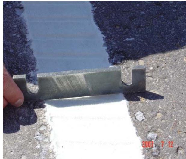
Template control, marking is flush with pavement
