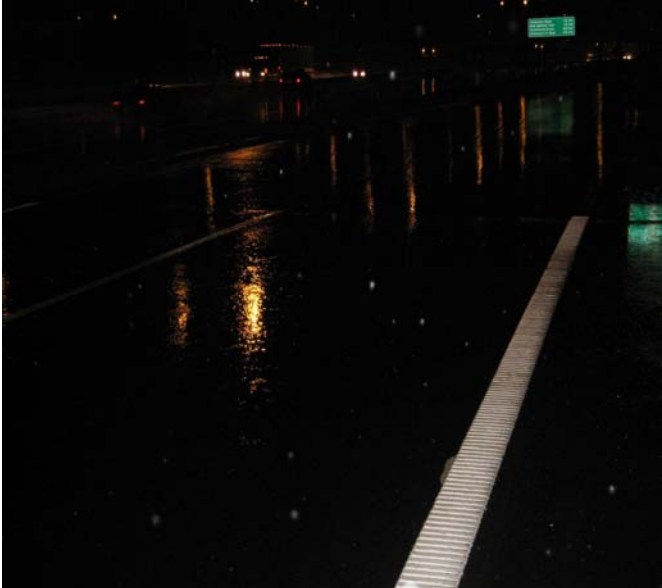
Rainline ends and paint begins; note that the paint lines are not visible during wet night conditions.
