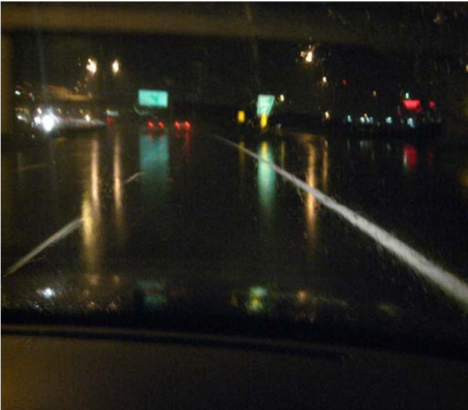
Rainline markings are visible during rain fall
