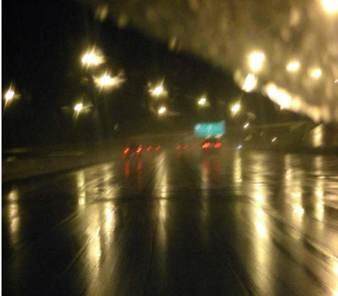
Paint lines not visible during rain fall
