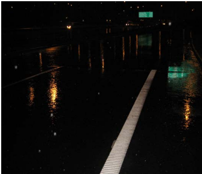
Rainline ends and paint begins; note that the paint lines are not visible during wet night conditions.
