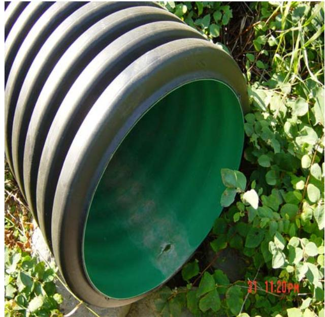
Soleno culvert (600mm diameter)
