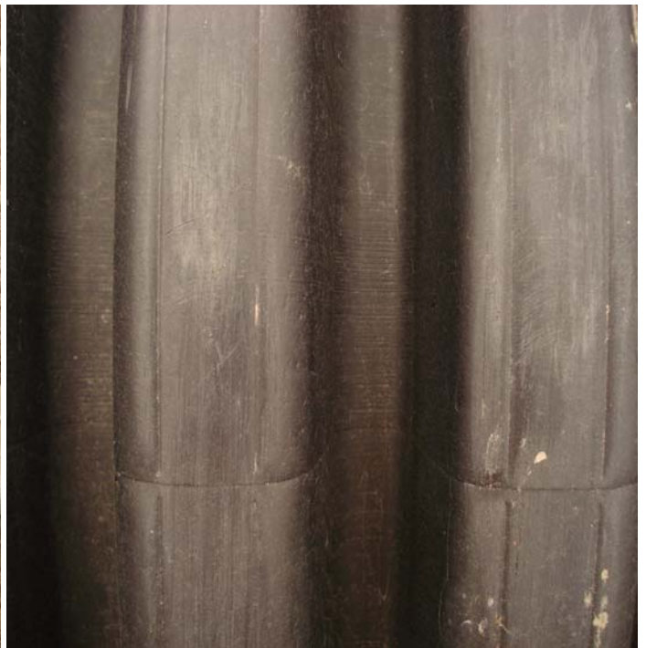
Close-up, no wall separation evident
