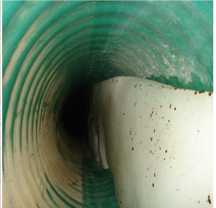
Interior of pipe
