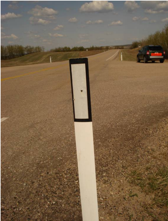
Steel-flex delineator in good shape
