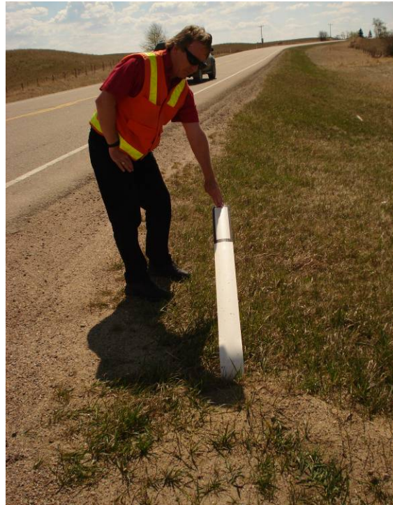
Delineator flex's when impacted and returns to original position
