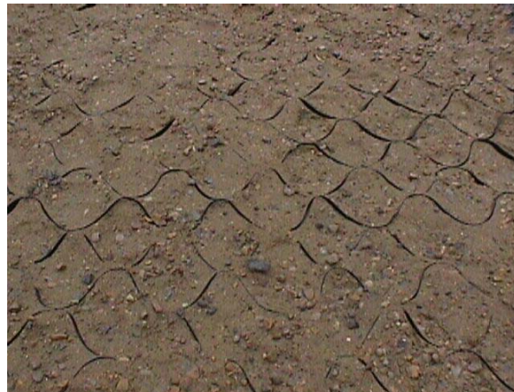
Geo-Cell – filled with gravel and sand and levelled
