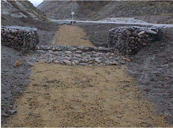
Geo-Cell (brown gravel) channel
