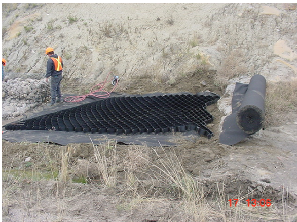
Geo-Cell webs are stretched and laid on geotextile
