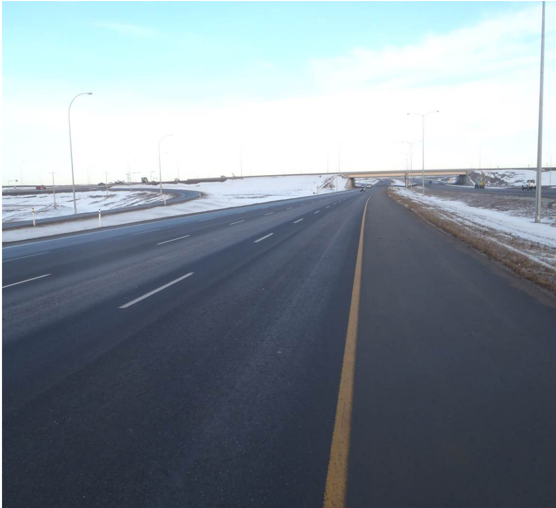
Overall view looking north
