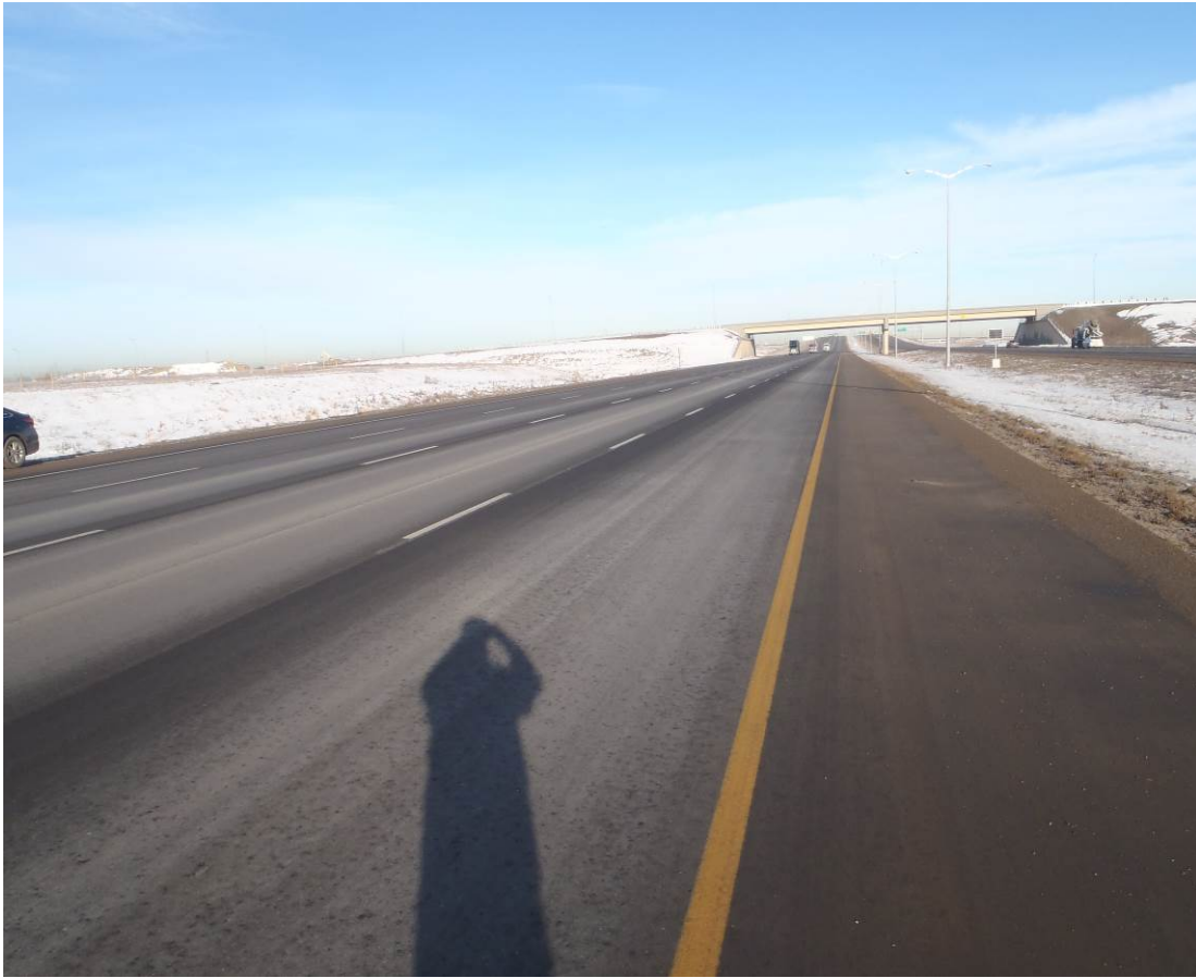
Overall view, looking north
