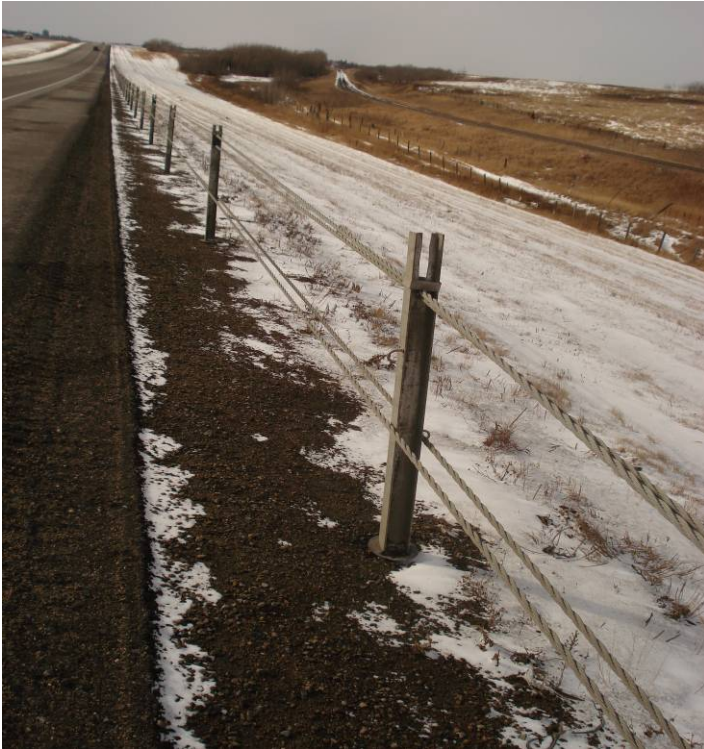
Cable is out of steel hooks
