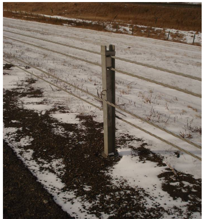
Cable is out of steel hooks
