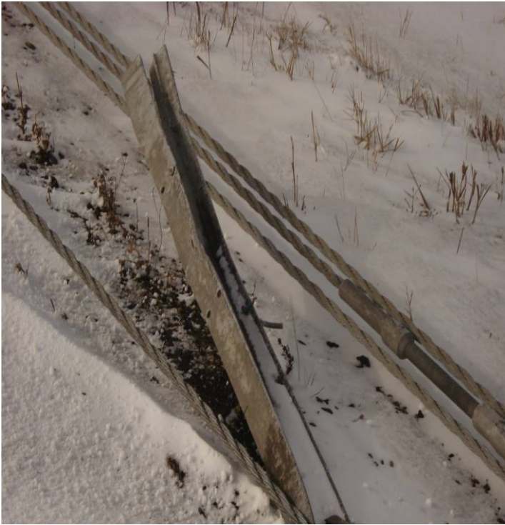
Cable lying on ground
