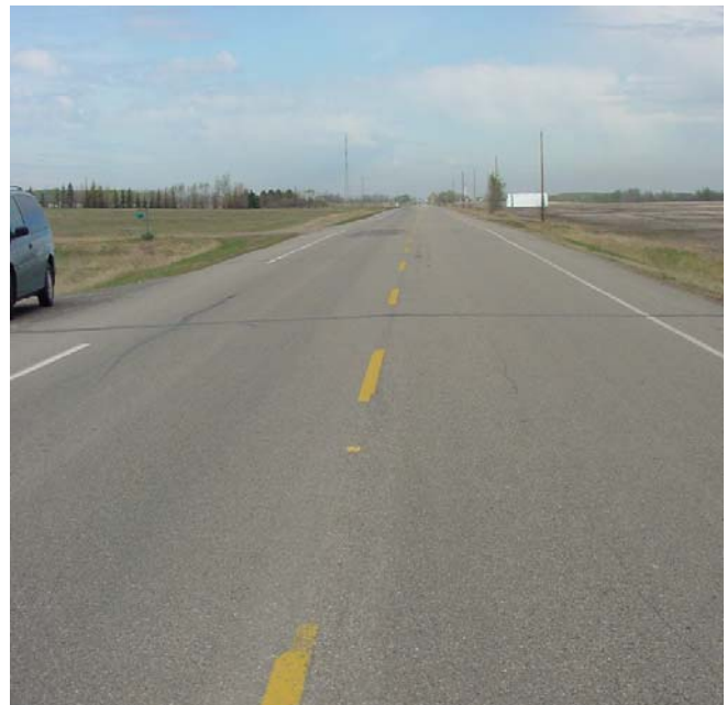
Alkyd paint lines, (looking west)
