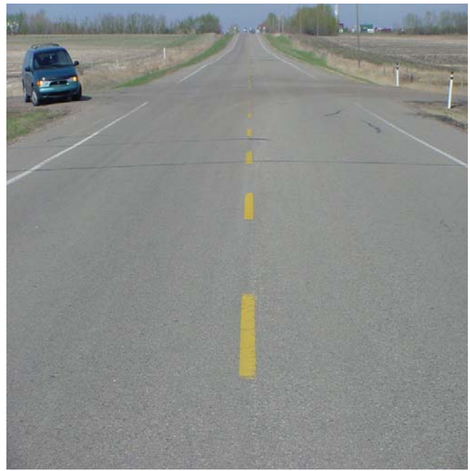
Alkyd centerline looking west
