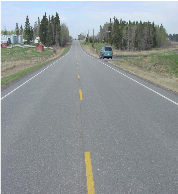
HD-21A paint lines, looking west
