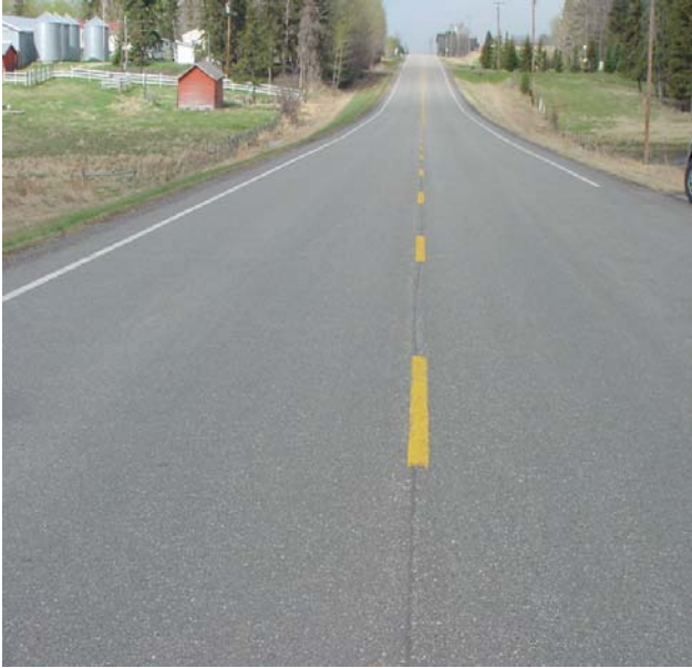
HD-21A paint lines, (looking west)
