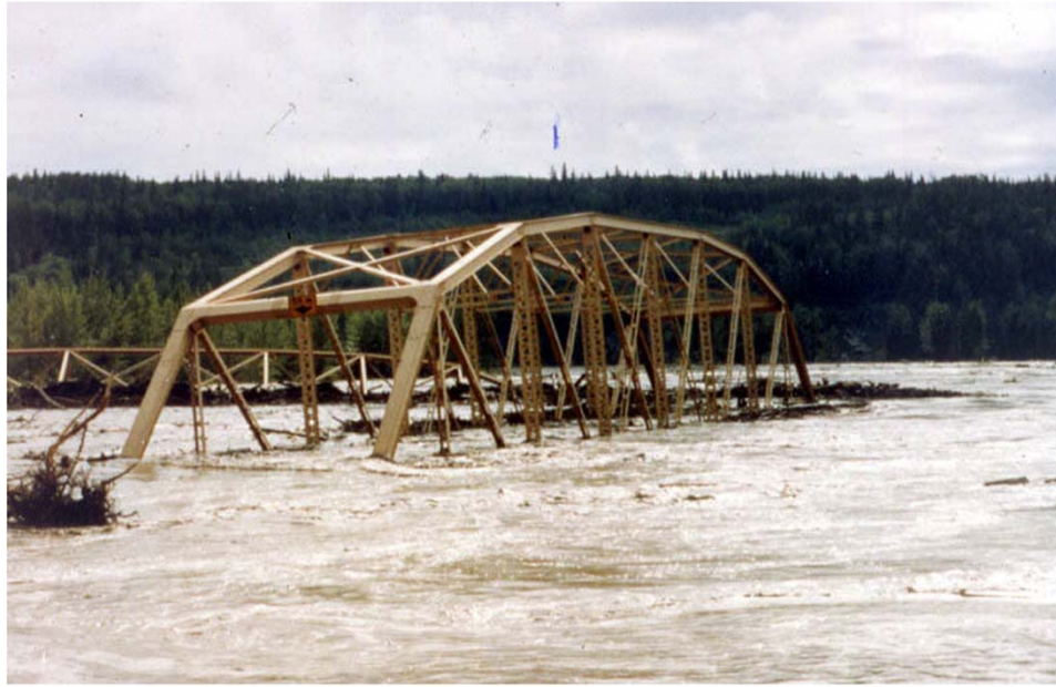
Superstructure carried away and damaged
