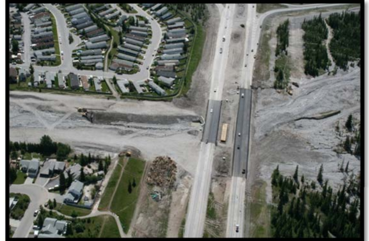
Post-repair at Cougar Creek
