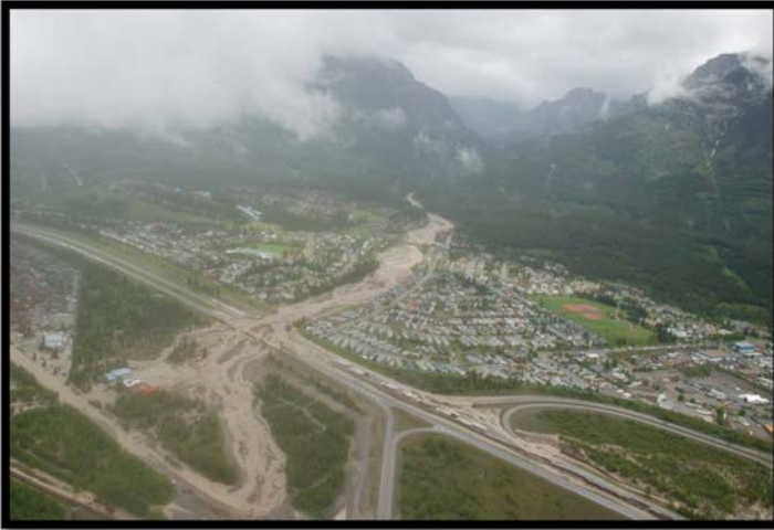
Flood damage at Cougar Creek
