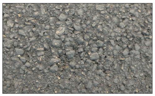
Photograph 9 - Moderate Segregation (bordering on Severe) (Close-Up)
