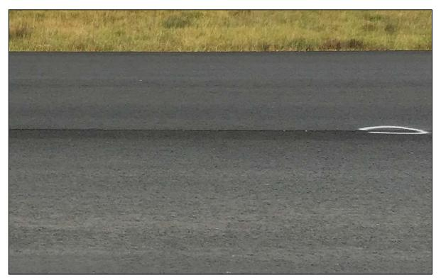
Photograph 15 - Improperly Matching Joint (View 2)
