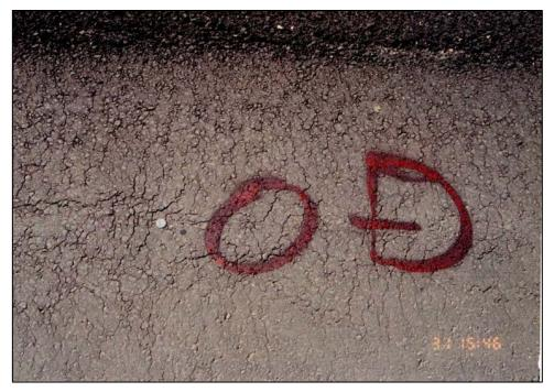
**Photograph 17 - Obvious Defect (Hairline Cracking)**
