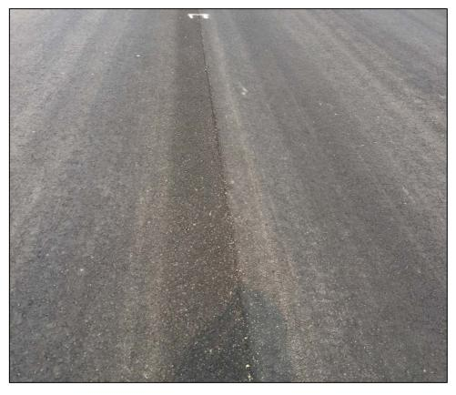
Photograph 14 - Improperly Matching Joint (View 1)
