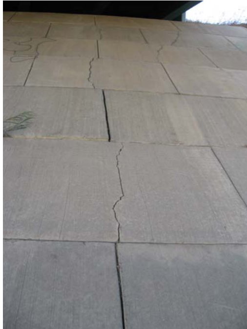
Photo 6 – Existing 17 Street NW bridge over Sherwood Park Freeway, north abutment. Cracks in the concrete panels of the head slope.
