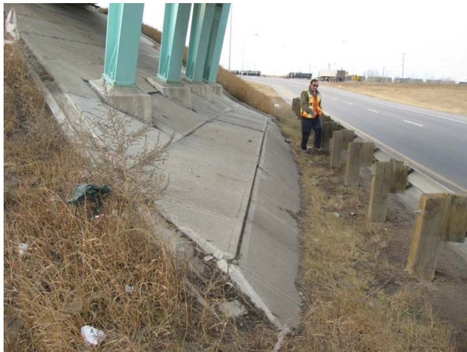
Photo 8 – Bulging observed in the lower part of the head slope at existing bridge (BF76649) northwest of proposed Bridge 23.
