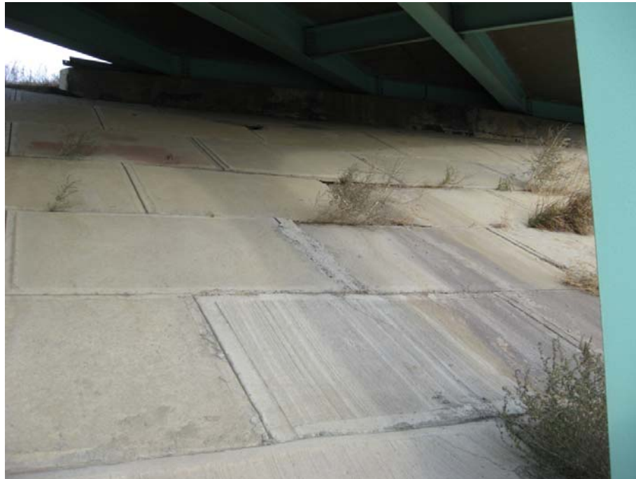
Photo 9 – Growing vegetation between concrete panels in the head slope at existing bridge (BF76649) northwest of proposed Bridge 23.
