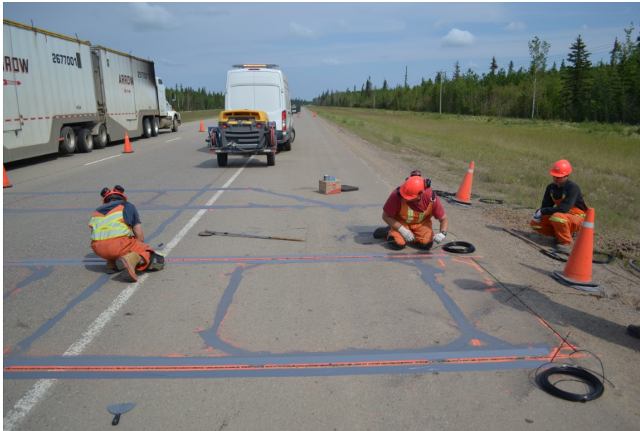
Figure 19: Weigh in Motion Installation on Pavement
