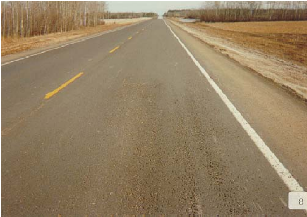
Photo Shows A Localized Area Of Pickouts Pickout Measurement Should NOT Occur In This Area
