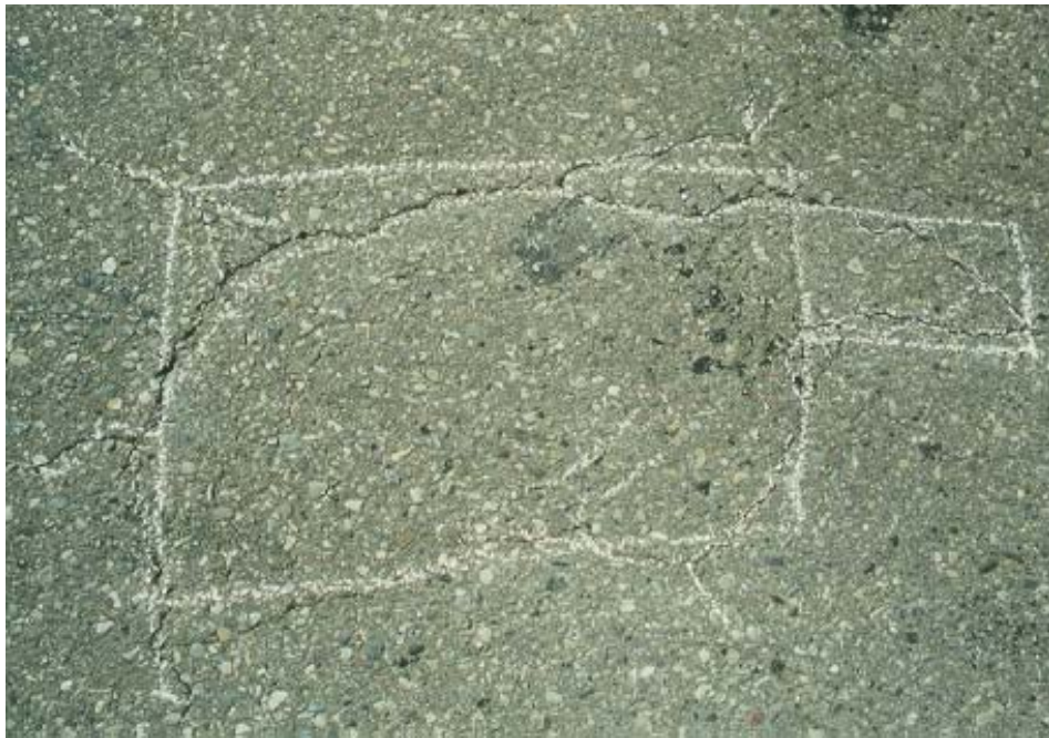
Chalked Area of Block Cracking
