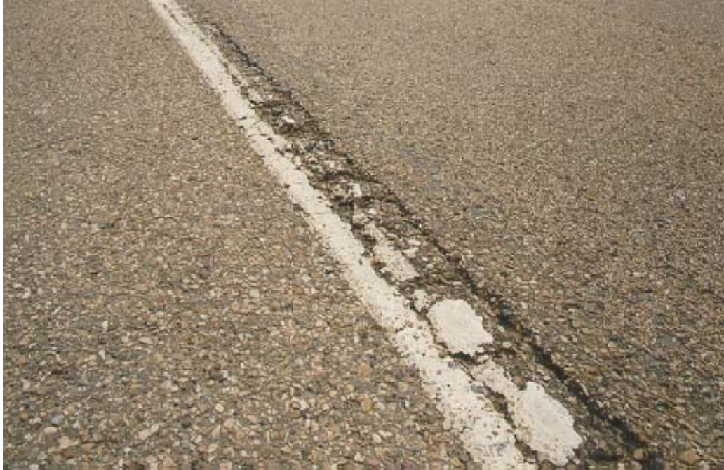
Extreme Ravelling To Be Recorded As A Surface Defect
