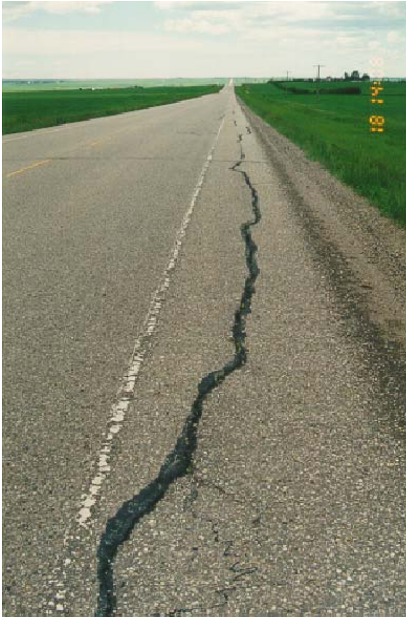
Longitudinal shoulder cracking
