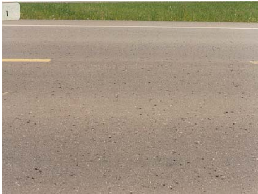
Pickouts Consistent Throughout Segment Good Location For Pickout Measurement
