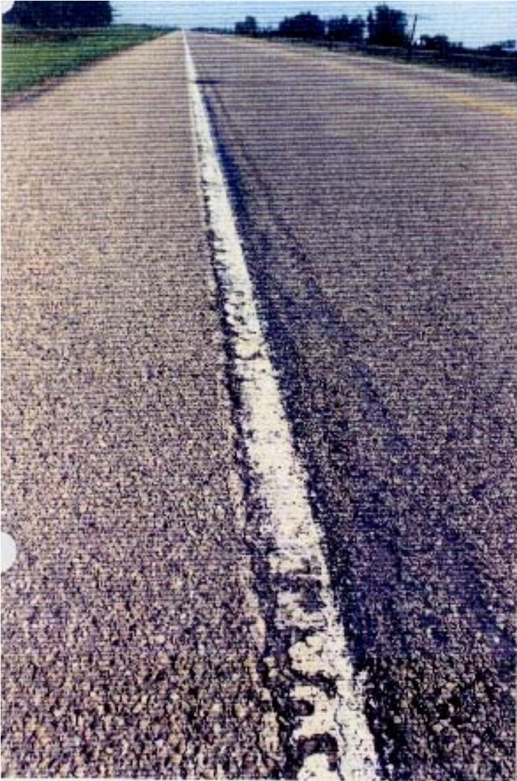
Extreme Ravelling To Be Recorded As A Surface Defect
