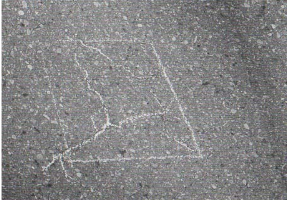
Area of Branched Cracking
