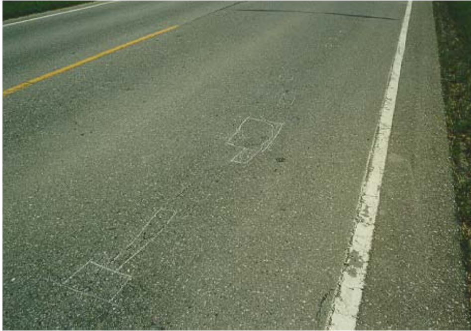
Areas of Block Cracking
