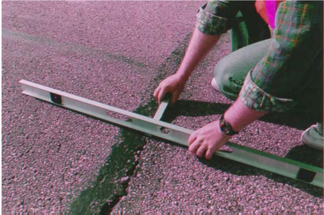
CORRECT - Obtain The Crack's Maximum Depression - Centre The Level Over The Crack And Measure The Depression At A Point Directly Over the Crack
