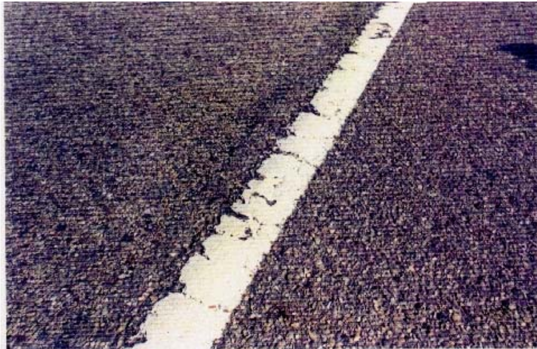
Area of Branched Cracking
