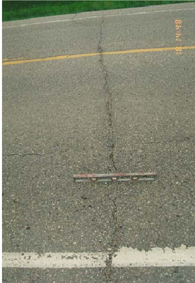
Severe transverse crack with a 4 mm dip and a centre of lane crack
