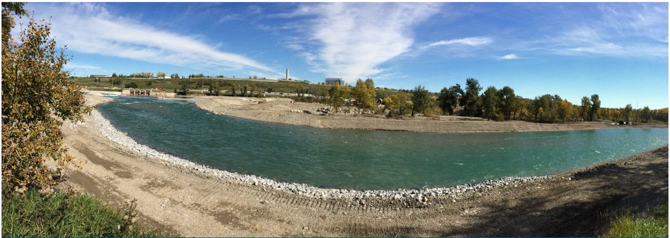
Temporary Bow River Diversion Channel (September 14, 2016)
