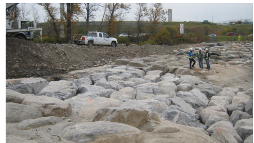
HWC Drop #3L Construction - September 30, 2016
