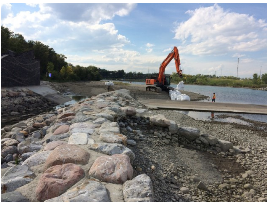
Cofferdam Construction - September 1, 2016
