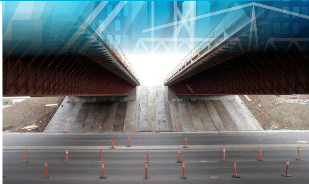
East embankment slope protection
