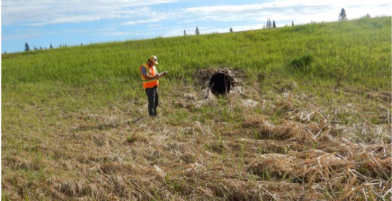
Photo No.5 – Outlet of SWSP culvert C2; minor flow observed in 2022
