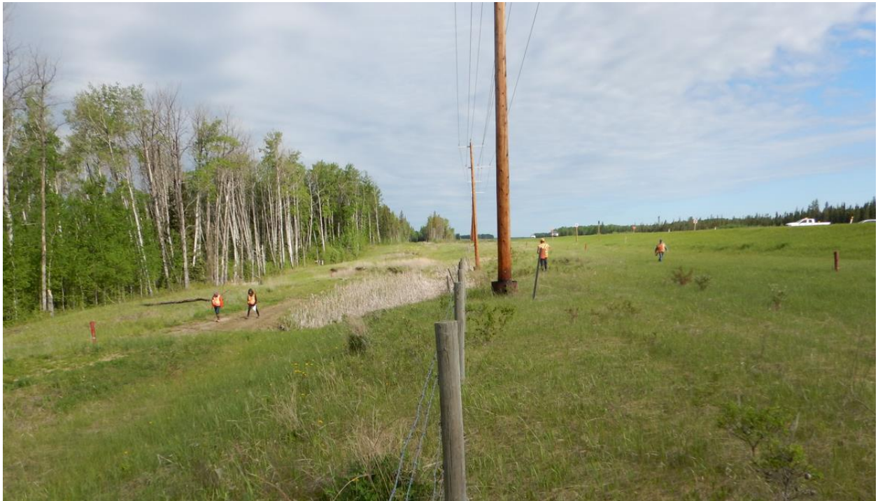
Photo No.4 – Looking north at the southern flank of upper and lower landslide blocks; note standing water within the flank and lateral shifting of existing fence; landslides are well vegetated
