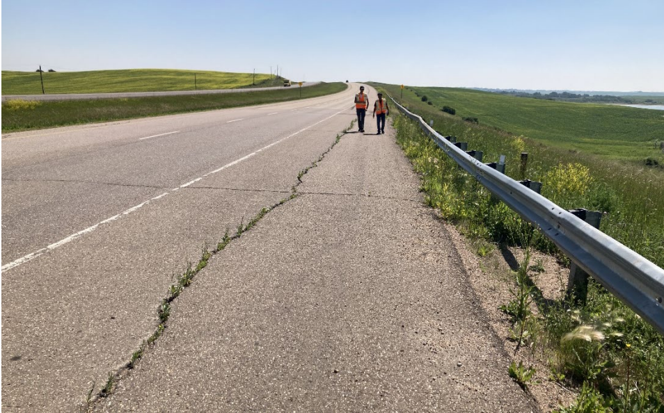
Photo 4 Ground settlement and cracking observed on the upper portion of the highway embankment slope downslope of the h-pile wall (crack indicated by red arrow). Photo taken June 28, 2023, facing north.
