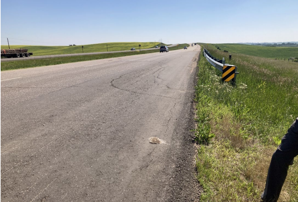
Photo 2 Asphalt cracking and settlement observed in the south (eastbound) lane. Asphalt cracking appears to have extended through a recent asphalt patch between 2020 and 2023. Photo taken June 28, 2023, facing west.
