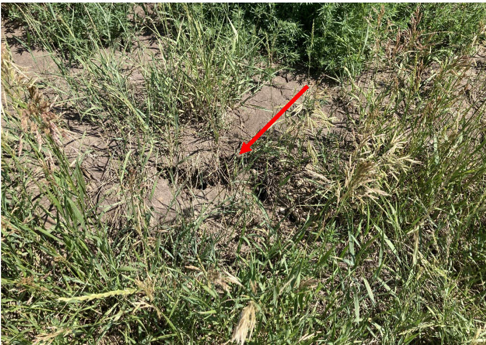
Photo 4 Ground settlement and cracking observed on the upper portion of the highway embankment slope downslope of the h-pile wall (crack indicated by red arrow). Photo taken June 28, 2023, facing north.
