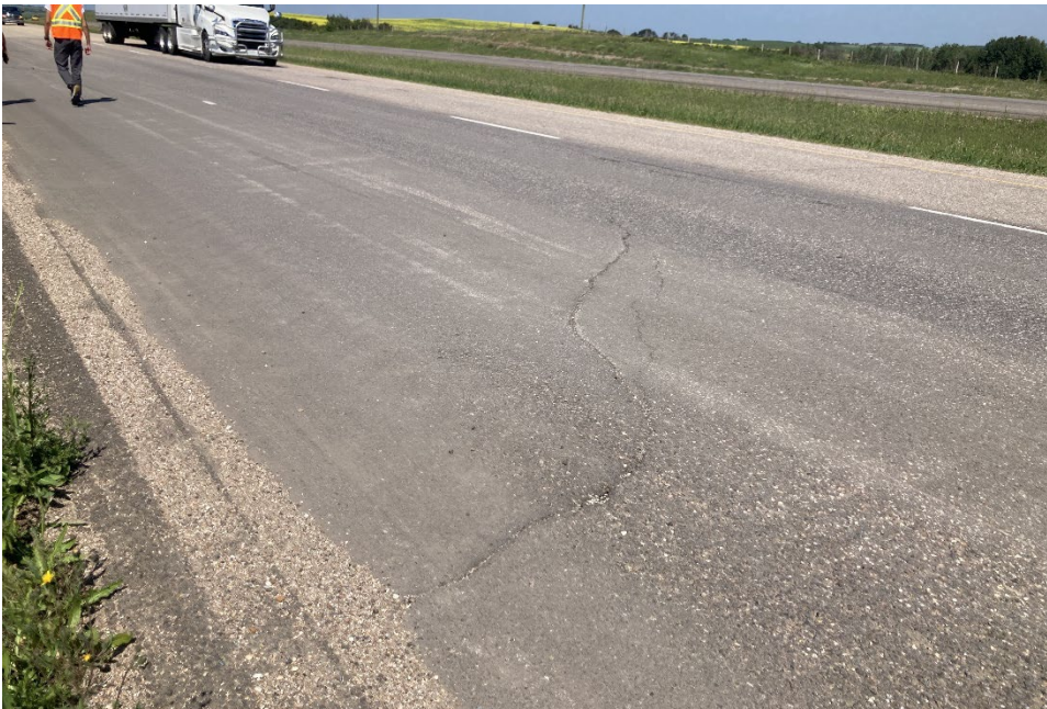
Photo 2 Asphalt cracking and settlement observed in the south (eastbound) lane. Asphalt cracking appears to have extended through a recent asphalt patch between 2020 and 2023. Photo taken June 28, 2023, facing west.
