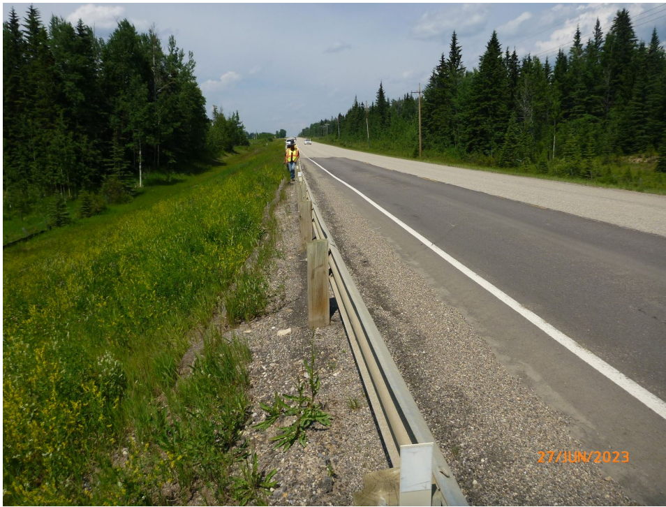
Photo 4 The repair of the highway embankment slope is well vegetated and appears to be performing well. Photo taken June 27, 2023, facing south.
