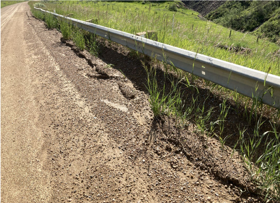
Photo 4 Head scarp of the slide where ground cracks were observed. Extent (number and width) of ground cracks have increased since the 2022 inspection. Photo taken June 18, 2024, facing east.
