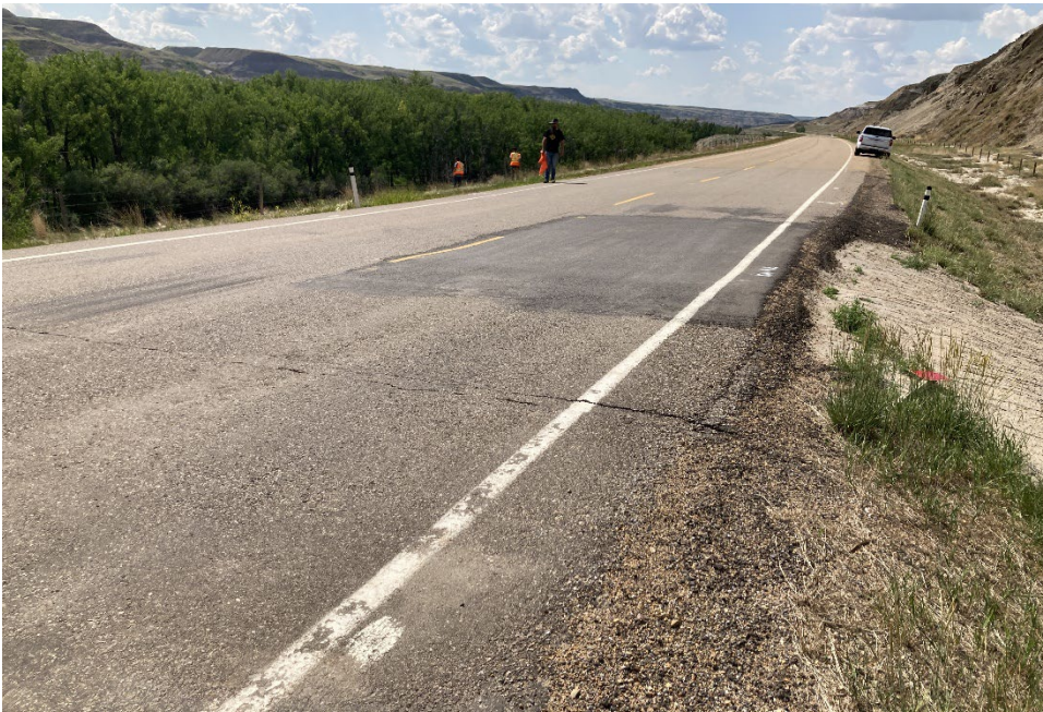
Photo 4 A pavement patch was completed in the north (westbound) lane at the C058-2 site between the 2021 and 2023 inspections in an area of previously observed settlement. Photo taken June 26, 2023, facing west.
