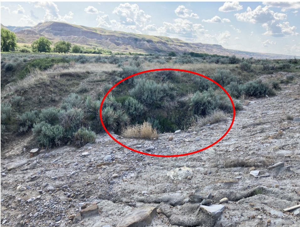
Photo 6 Large sinkhole (indicated by a red circle) at the toe of the south highway embankment at C058-3 appears to have expanded since the 2021 inspection. Photo taken June 26, 2023, facing southwest.
