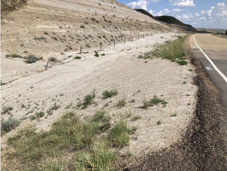
Photo 4 A pavement patch was completed in the north (westbound) lane at the C058-2 site between the 2021 and 2023 inspections in an area of previously observed settlement. Photo taken June 26, 2023, facing west.
