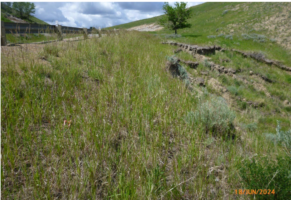
Photo 3 Ground cracking between 1 m to 1.5 m upslope of the head scarp (within 3 m of the guardrail) was observed during the 2024 inspection. Photo taken June 18, 2024, facing west.
