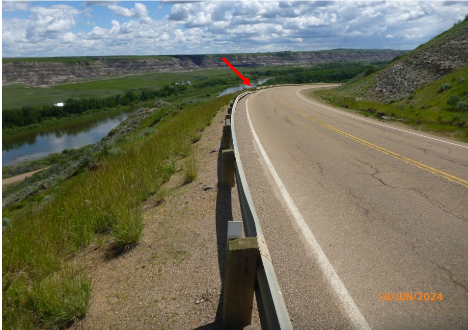
Photo 7 The erosion in the south (eastbound) lane near the midpoint of the C017-2 site is expanding and it within 2 m of the edge of pavement. Photo taken June 18, 2024, facing east.
