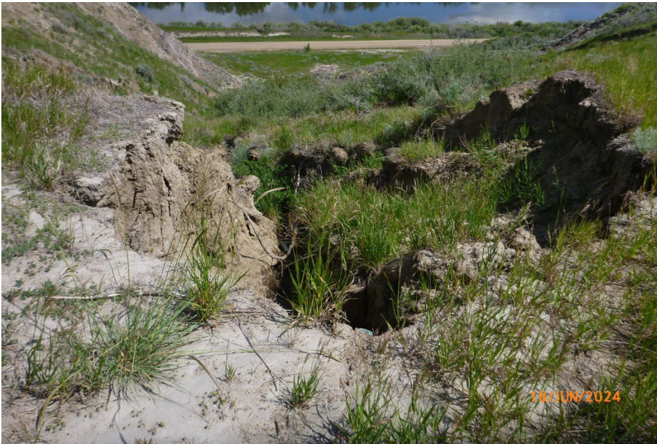
Photo 3 Ground cracking between 1 m to 1.5 m upslope of the head scarp (within 3 m of the guardrail) was observed during the 2024 inspection. Photo taken June 18, 2024, facing west.
