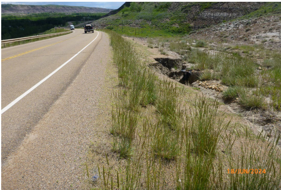
Photo 7 The erosion in the south (eastbound) lane near the midpoint of the C017-2 site is expanding and it within 2 m of the edge of pavement. Photo taken June 18, 2024, facing east.
