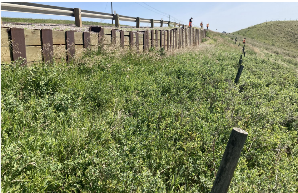
Photo 2 Timber lagging and west h-pile wall extension installation completed in early-2021. Photo taken June 26, 2023, facing east.
