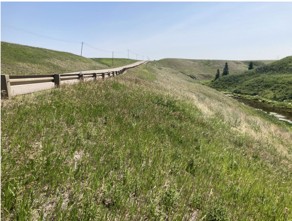
Photo 6 The vegetation coverage at the C048-3 slide repair (completed fall of 2020) has improved since the 2021 inspection. Photo taken June 26, 2023, facing east.
