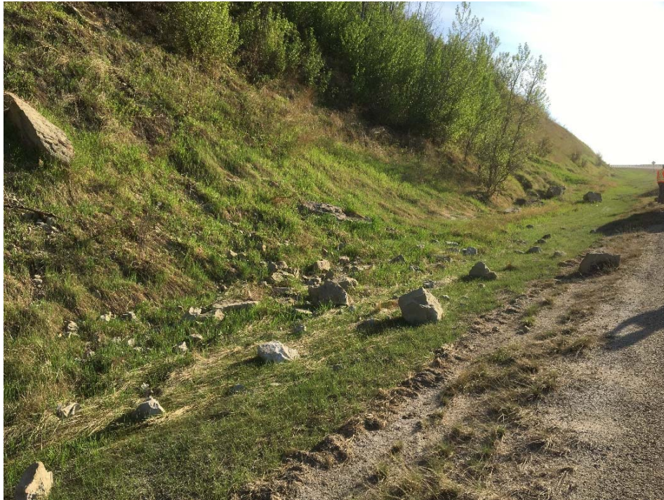
Photo 1: Looking northeast from the SBL shoulder at km 12.32 of Hwy 2:68 at sandstone blocks in the ditch and along the sideslope above the highway.
