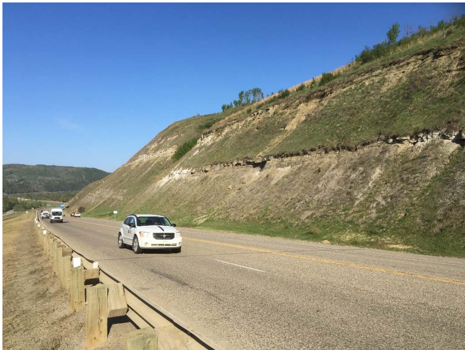
Photo 9: Looking NW from the guardrail at km 12.46 west of the debris flow at salt staining/soil loss below the lower sandstone ledge and an erosion gully in the backslope (May 15, 2018)
