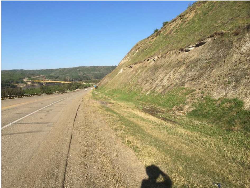
Photo 8: Looking southwest from the shoulder of the SBL at km 12.435 along the SBL at the staining in the backslope and the soil loss below the lower sandstone ledge.
