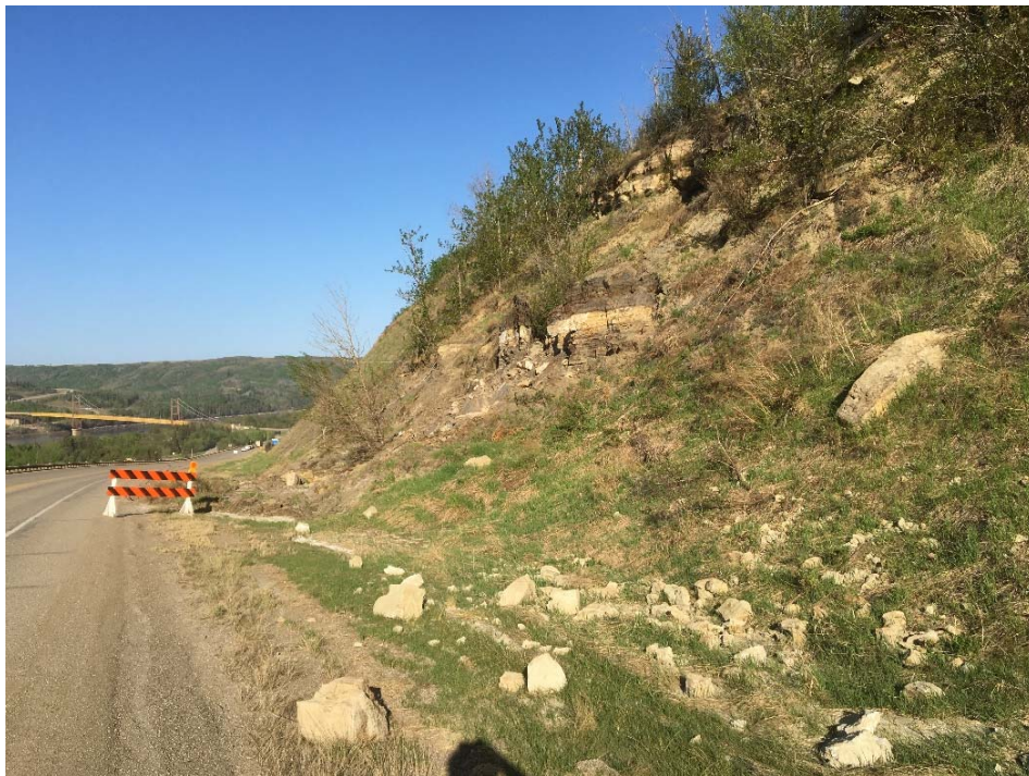
Photo 2: Looking southwest from the shoulder of the SBL from km 12.29 of Hwy 2:68 at the accumulated debris and sandstone pieces along the base of the debris flow.
