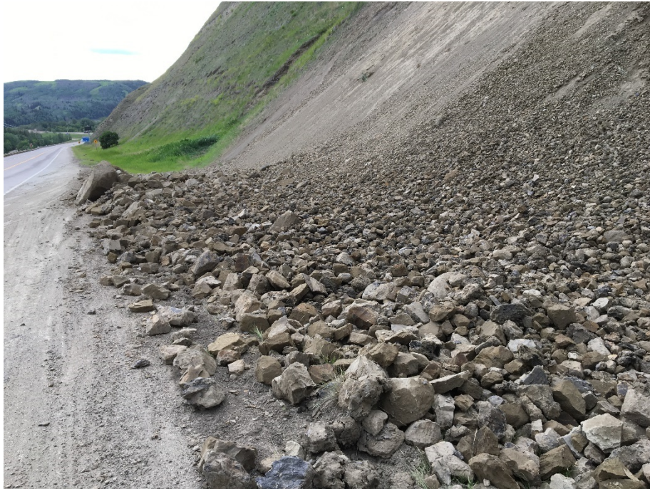
Photo 5: Looking west from SBL ditch of Hwy 2:68 at sandstone slabs and soil chunks that have accumulated in the ditch below the landslide (June 26, 2018)
