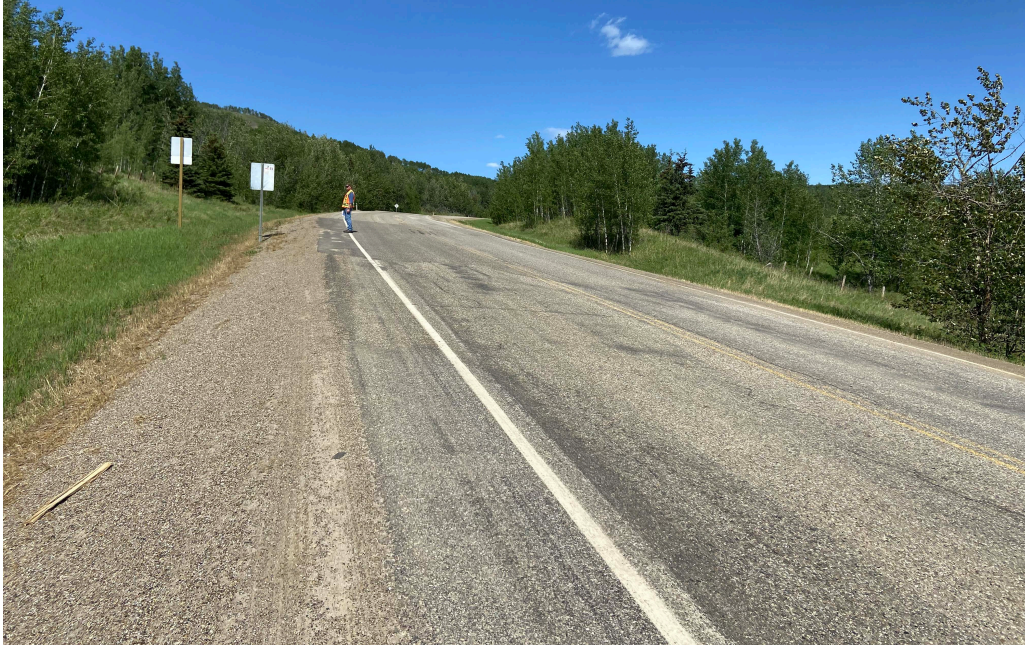
Photo 5 – Looking east where the slide scarp crosses the highway at the east end of the site and ACP patch.
