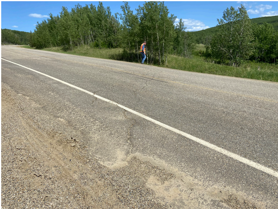
Photo 6 – Looking southeast at the scarp crack reflecting through the ACP patch placed over the east end of the site.
