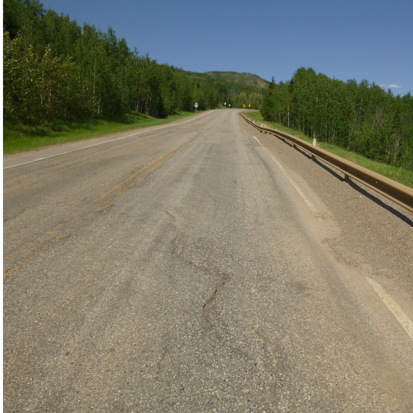
Photo 1 – Looking east along the cracked highway surface from the west end of the site. Note the west dip in the road/guardrail.
