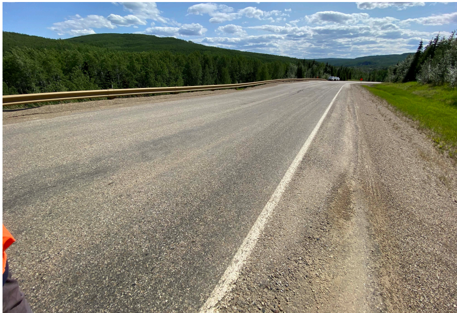
Photo 4 - Looking west at the dip/sunken highway where the slide scarp crosses the west end of the site.
