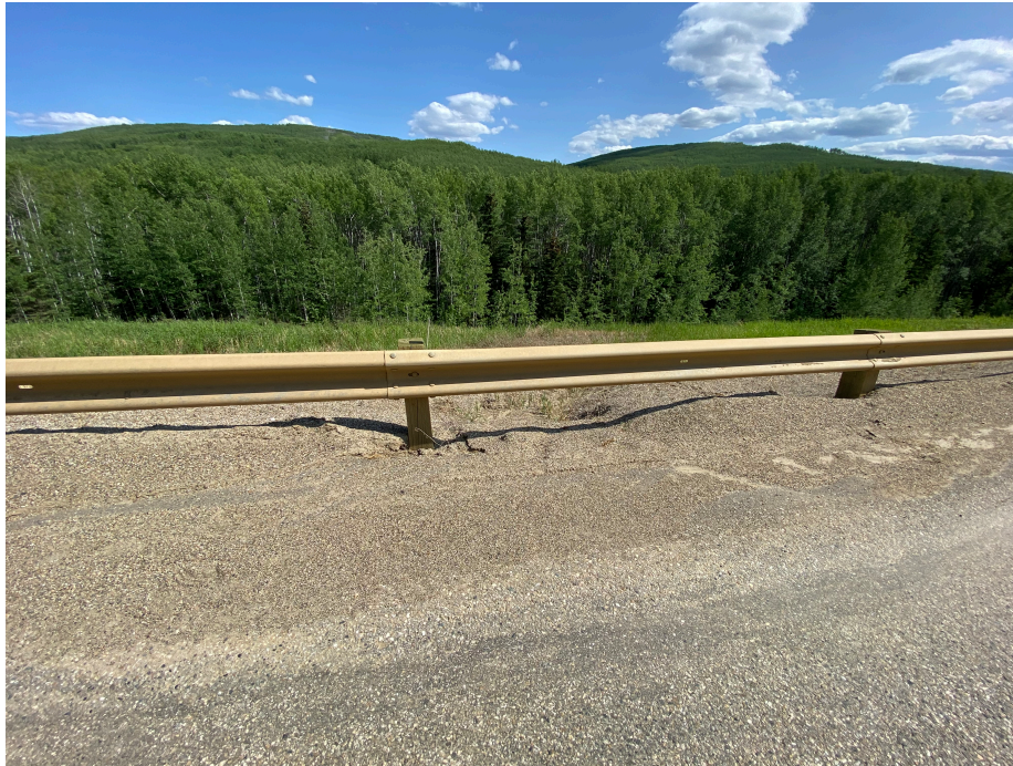
Photo 3 - Looking south where channelized surface runoff flowing along the dip in the highway has breached the sand build-up underneath the south guardrail and created an erosion gully in the hwy embankment slope below.
