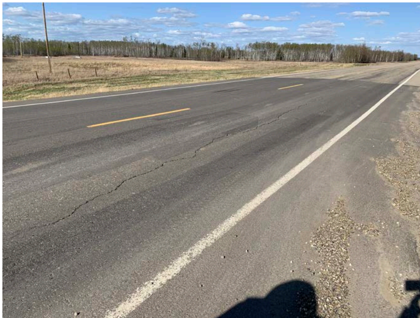
Photo 4 – Looking northeast along the highway at the cracks west of and over the culvert adjacent to the East Slide.
