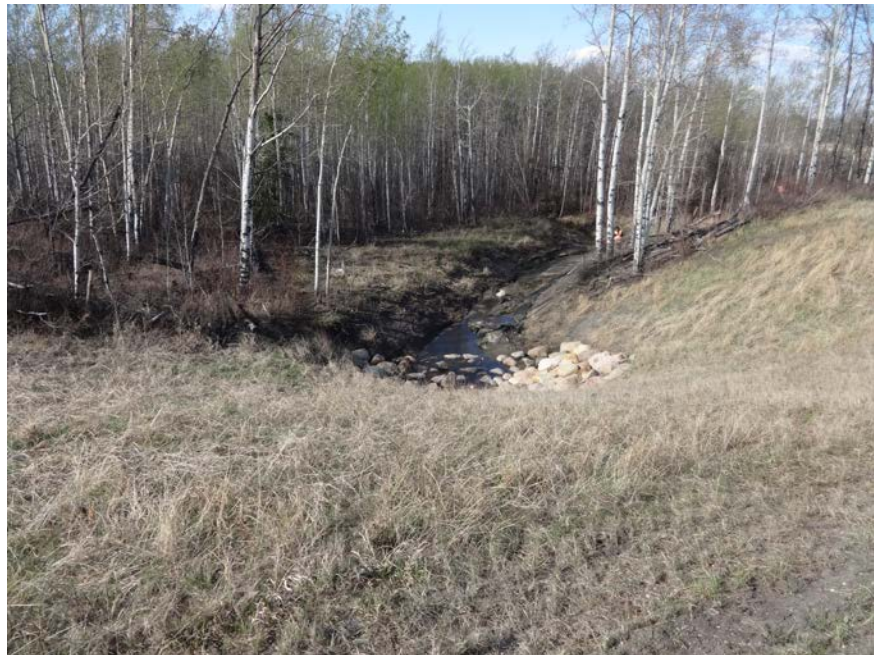
Photo 2 – Looking northeast at the highway embankment, culvert outlet and extended channel over/beyond the West Slide.
