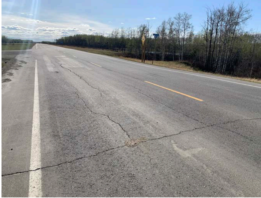
Photo 3 – Looking west along the highway from the 900 mm SWSP culvert crossing the highway of the East Slide. A few cracks have formed through the new pavement surface placed in 2022, west of and overtop of this culvert.
