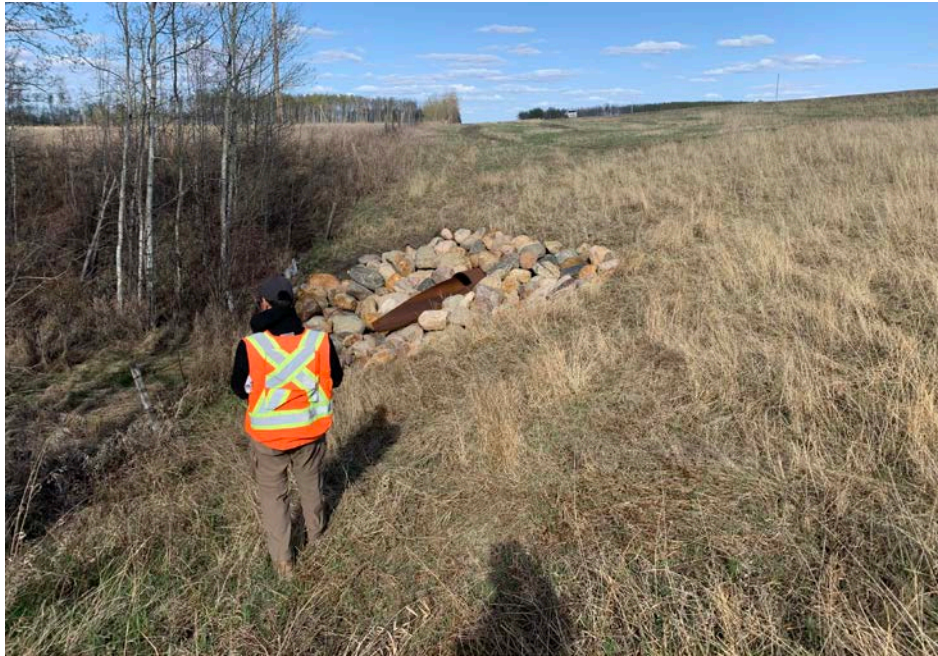
Photo 5 – Looking east at the 900 mm dia. SWSP outlet and north downstream embankment of the East Slide.
