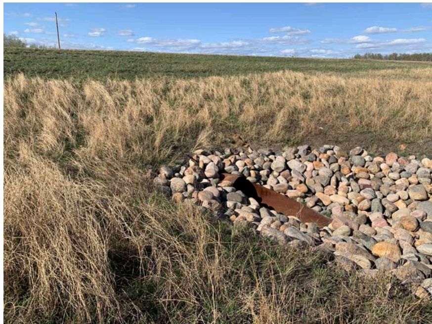
Photo 6 – Looking southeast across the 900 mm SWSP inlet of the East Slide.
