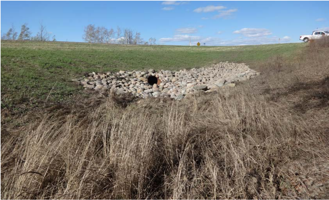
Photo 1 – Looking northeast across the culvert inlet area and channel riprap of the West Slide.
