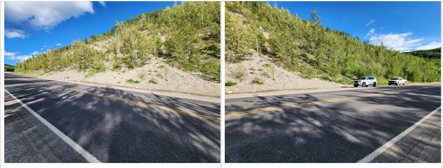
Photo 1 Pavement surface and backslope on east side of Hwy 40:34. Note areas of poor vegetation, exposed gravelly material, and gully and rill erosion on backslope. Photo taken June 10, 2024, facing northeast and southeast, respectively.
