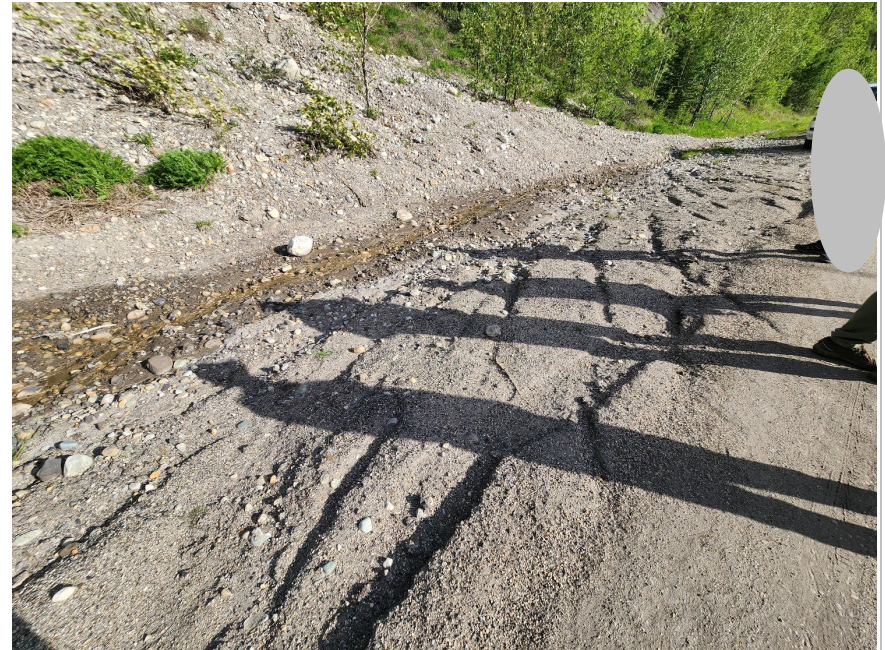
Photo 2 Water flowing in ditch at toe of backslope on east side of Hwy 40:34. Photo taken June 10, 2024, facing northeast and southeast, respectively.
