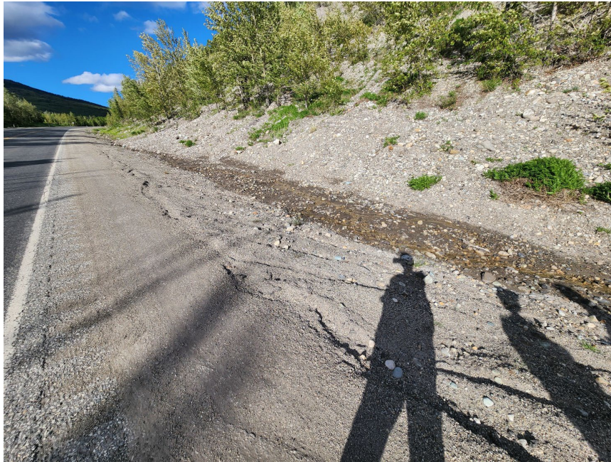
Photo 2 Water flowing in ditch at toe of backslope on east side of Hwy 40:34. Photo taken June 10, 2024, facing northeast and southeast, respectively.
