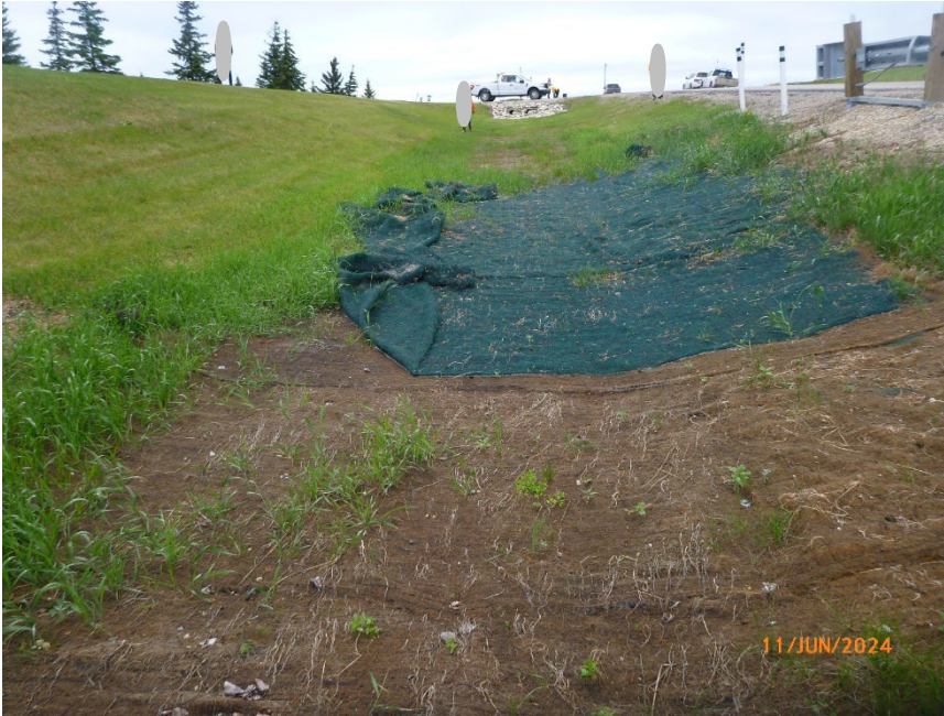
Photo 9 Unarmoured ditch on west side of Hwy 724:04. Photo taken June 11, 2024, facing southwest.
