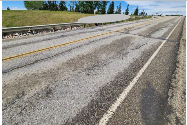
Photo 11 Pavement surface of Hwy 724:04. Some cracking above the previously repaired erosion gully. Photos taken June 11, 2024, facing southwest and northwest, respectively.
