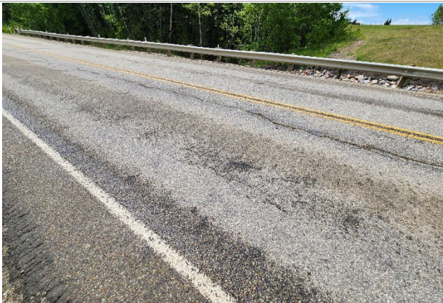
Photo 11 Pavement surface of Hwy 724:04. Some cracking above the previously repaired erosion gully. Photos taken June 11, 2024, facing southwest and northwest, respectively.
