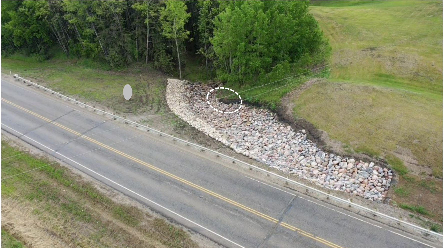
Photo 3 Riprap-lined channel constructed in 2023 in former erosion gully. Note riprap a little low on inside corner (circled in white). Photo taken with UAV June 11, 2024, facing southwest.
