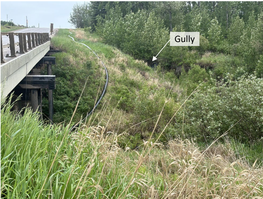
Photo 13 West side of Hwy 724:04 and bridge at GP039-II site. Note erosion gully (see next photo). Photo taken June 11, 2024, facing south from north abutment of bridge.
