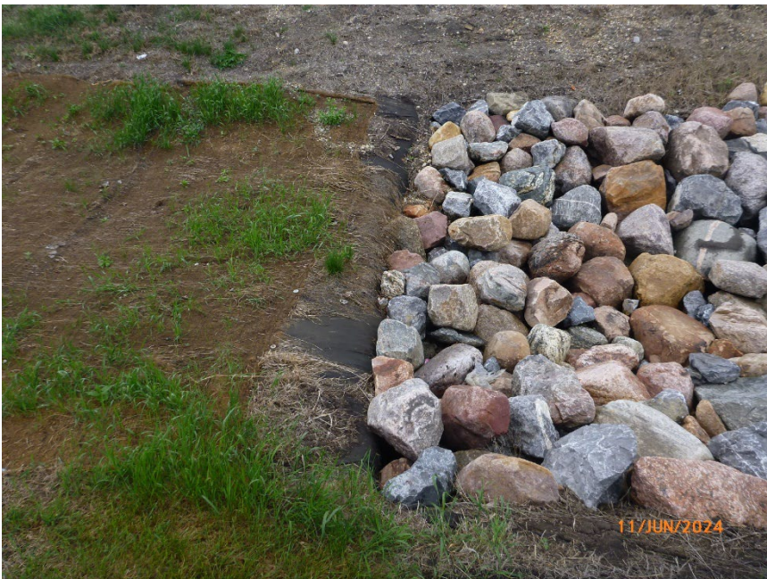
Photo 7 Transition between unarmoured ditch and riprap-lined channel. and Photo taken June 11, 2024, facing east.
