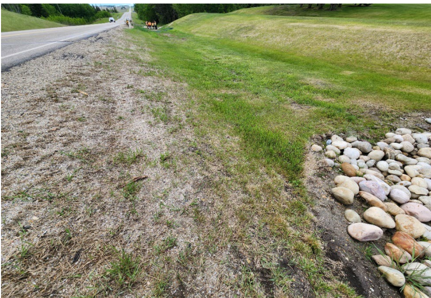
Photo 9 Unarmoured ditch on west side of Hwy 724:04. Photo taken June 11, 2024, facing southwest.
