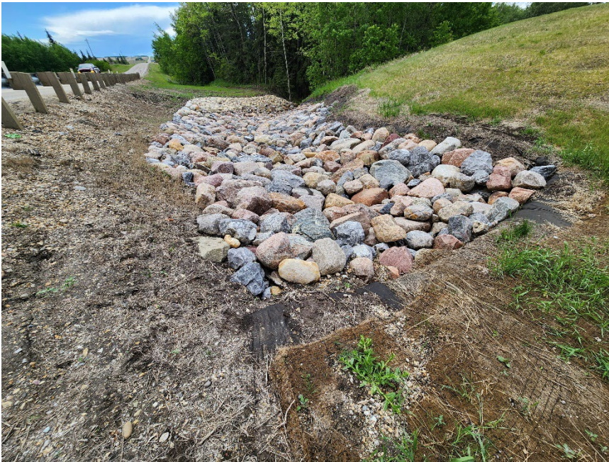
Photo 7 Transition between unarmoured ditch and riprap-lined channel. and Photo taken June 11, 2024, facing east.
