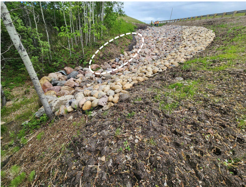
Photo 5 End of riprap-lined channel. Note riprap a little low on inside corner (circled in white). Photo taken June 11, 2024, facing northeast.
