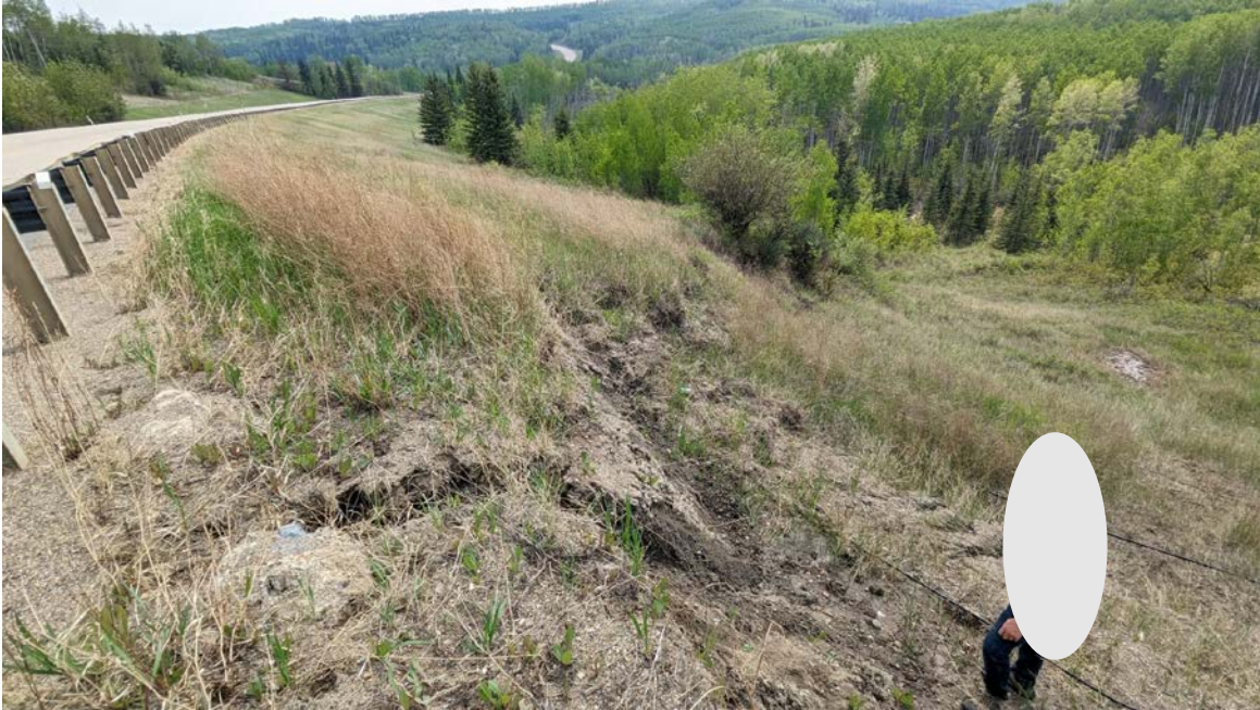
Photo 3 – Slide B: Looking south at the south half of the backscarp including two recently-exposed piles in the foreground near the guardrail.
