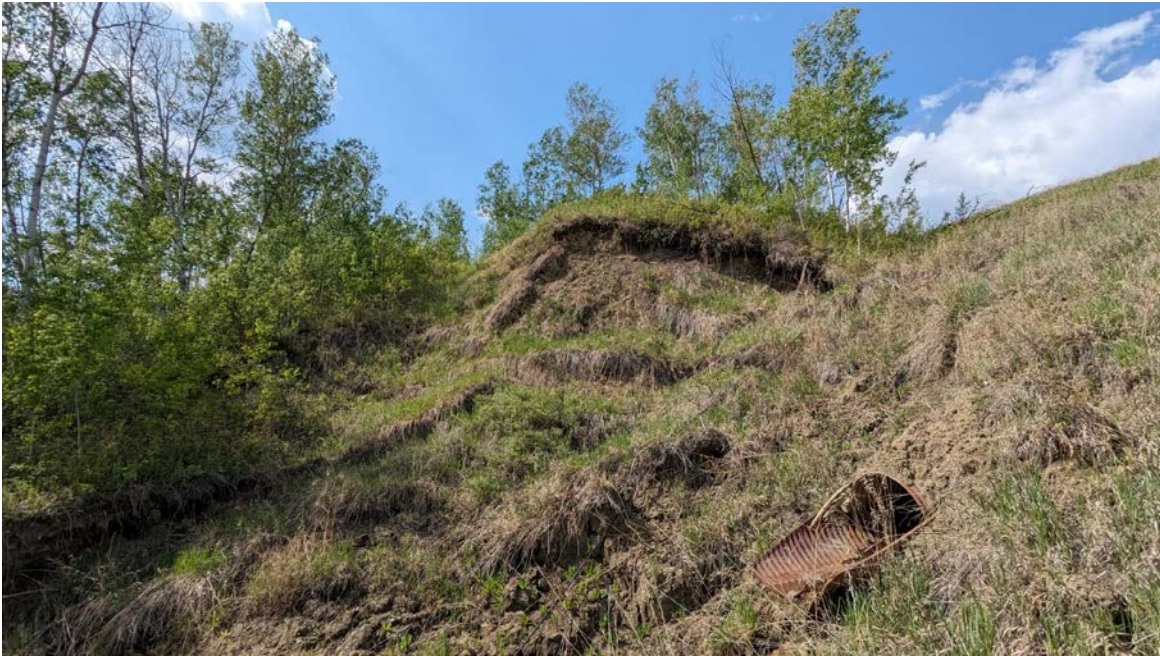
Photo 9 – Slide A: Looking northwest across hanging culvert outlet and knoll beyond where some vegetation has slumped off the face.
