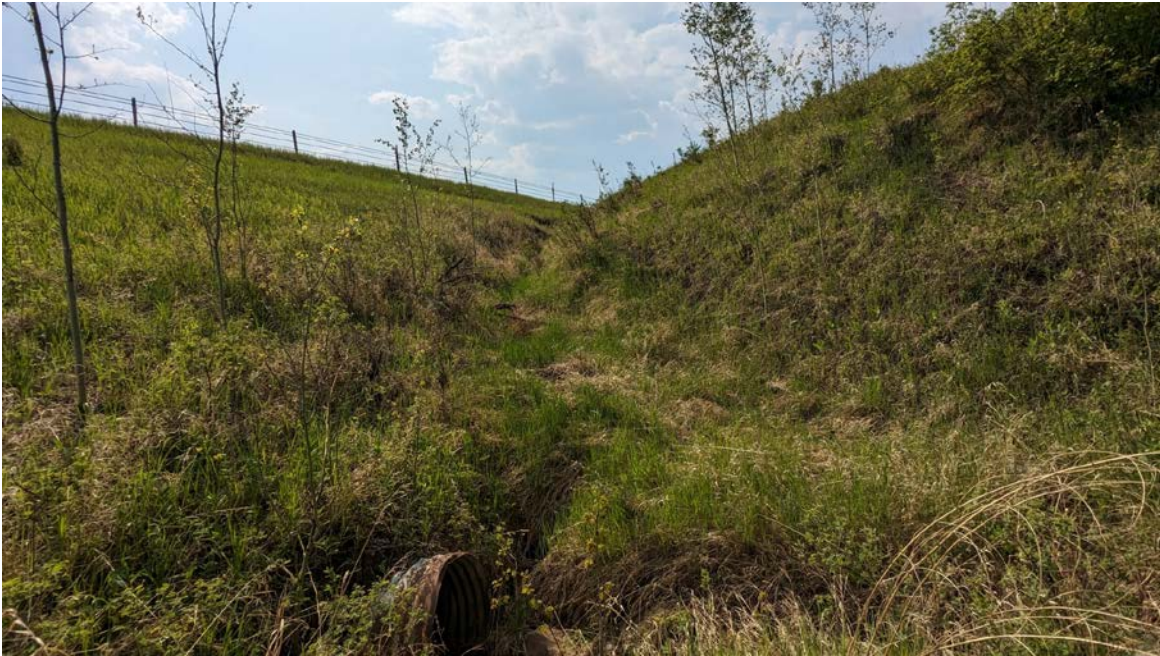
Photo 11 – Slide A: Looking north at an erosion gully in sideslope draining towards culvert inlet.
