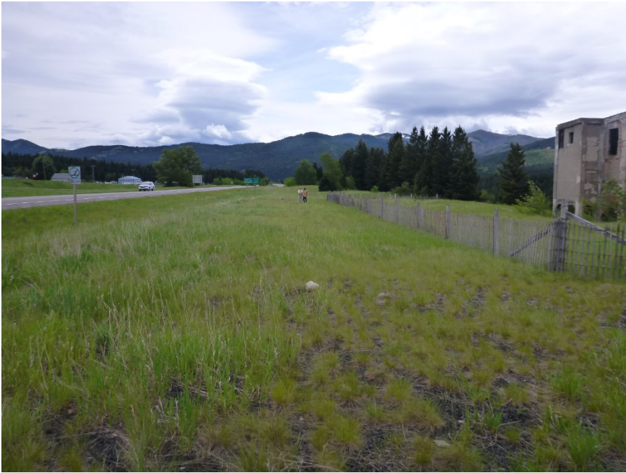
Photo 2 Sinkhole filled in due to collapse of old coal mine workings with old coal mining building in background. Photo taken facing west on June 1, 2017.
