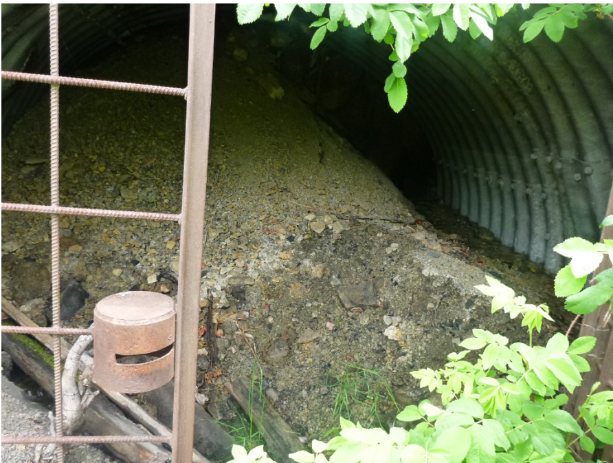
Photo 4 Mine-collapse debris inside old mine shaft. Ground water seepage exiting shaft. Photo taken facing north on June 1, 2017.
