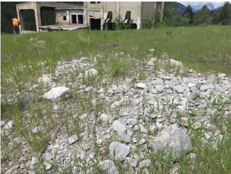
Photo 2 Sinkhole filled in due to collapse of old coal mine workings with old coal mining building in background. Photo taken facing west on June 1, 2017.
