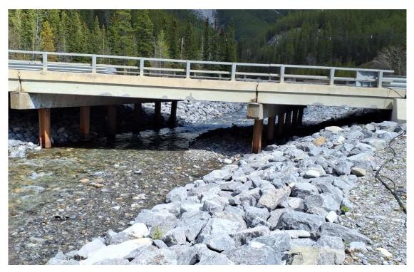
Photo 2 Upstream side of Rocky Creek Bridge. The upstream H-piles appear partially displaced from a suspected high-water event. Photo taken May 27, 2024, facing north.
