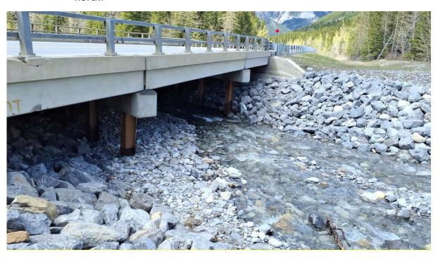
Photo 3 Upstream pile on north side of bridge. Pile looks to be displaced, but also could have been installed with some batter due to an obstruction during installation. Photo taken May 27, 2024, facing north.
