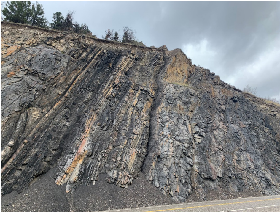
Photo 2 Erosion of soil at brow of slope leading to rockfalls and debris fans in the ditch. Note large boulders at crest of slope. Photo was taken facing northwest on May 9, 2023.
