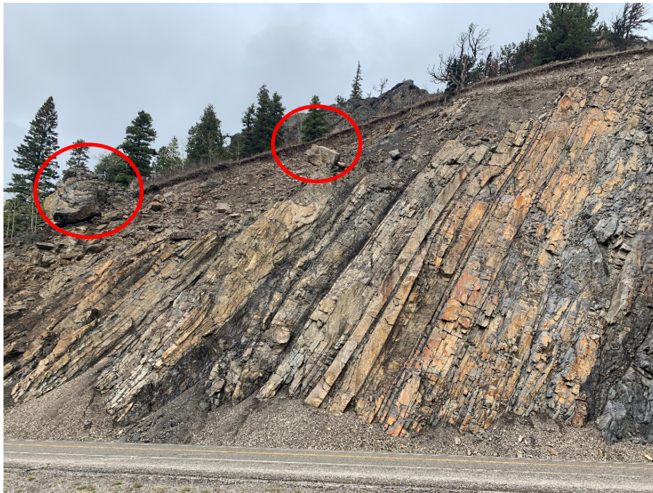
Photo 2 Erosion of soil at brow of slope leading to rockfalls and debris fans in the ditch. Note large boulders at crest of slope. Photo was taken facing northwest on May 9, 2023.
