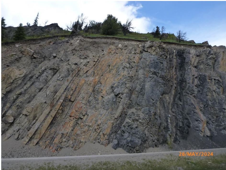
Photo 2 Erosion of soil at brow of slope leading to rockfalls and debris fans in the ditch. Note large boulders at crest of slope. Photo was taken facing north on May 28, 2024.
