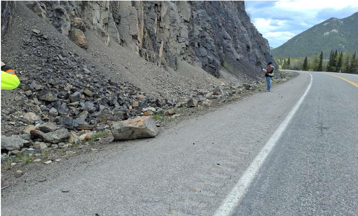
Photo 3 Active rockfall - debris fans and large rocks in ditch. The ditch should be regularly cleaned of debris. Photo taken facing east on May 28, 2024.
