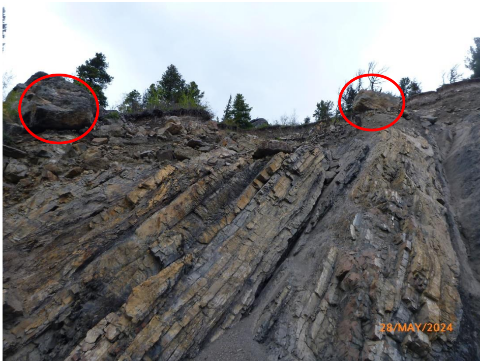
Photo 2 Erosion of soil at brow of slope leading to rockfalls and debris fans in the ditch. Note large boulders at crest of slope. Photo was taken facing north on May 28, 2024.
