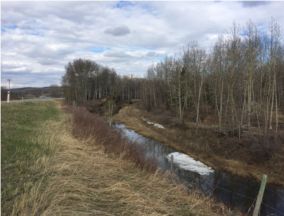
Photo 2 Downstream of eroded slope. No change in creek erosion towards road embankment in approximately 5 years. Photo was taken facing northeast on May 1, 2018.
