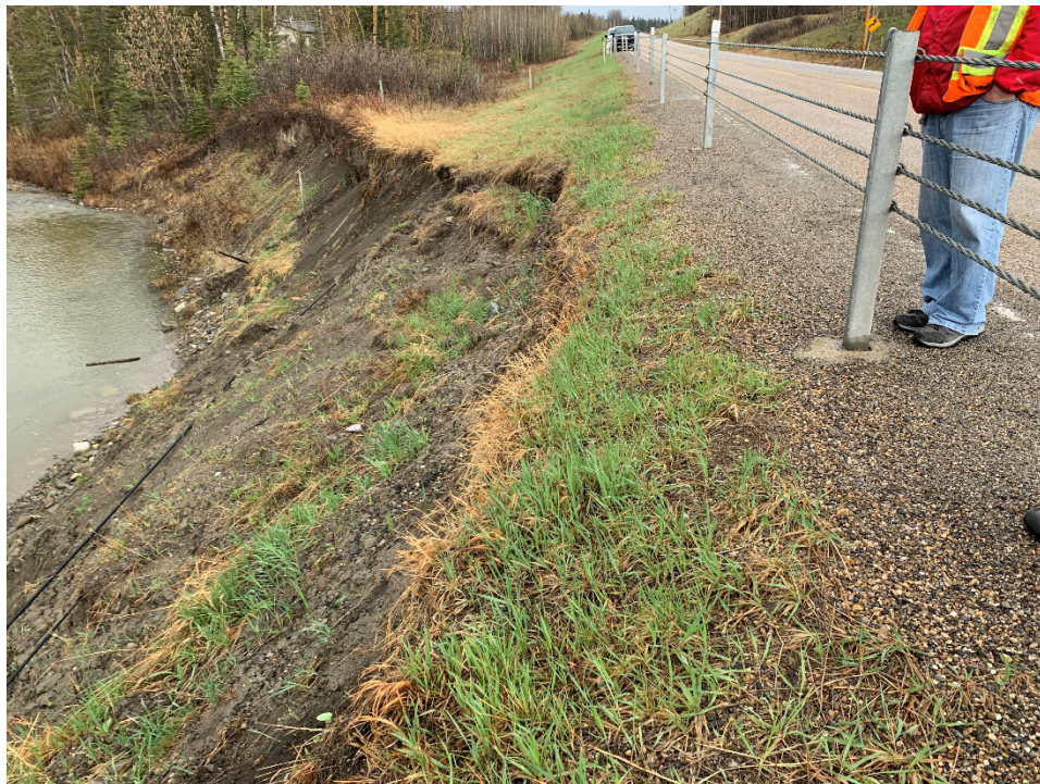
Photo 4 Crest of erosion approximately 1.1 m from guardrail. Photo taken facing west on May 9, 2023.
