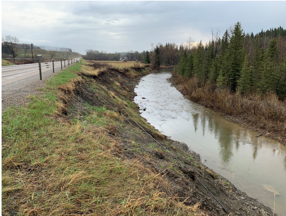
Photo 4 Crest of erosion approximately 1.1 m from guardrail. Photo taken facing west on May 9, 2023.
