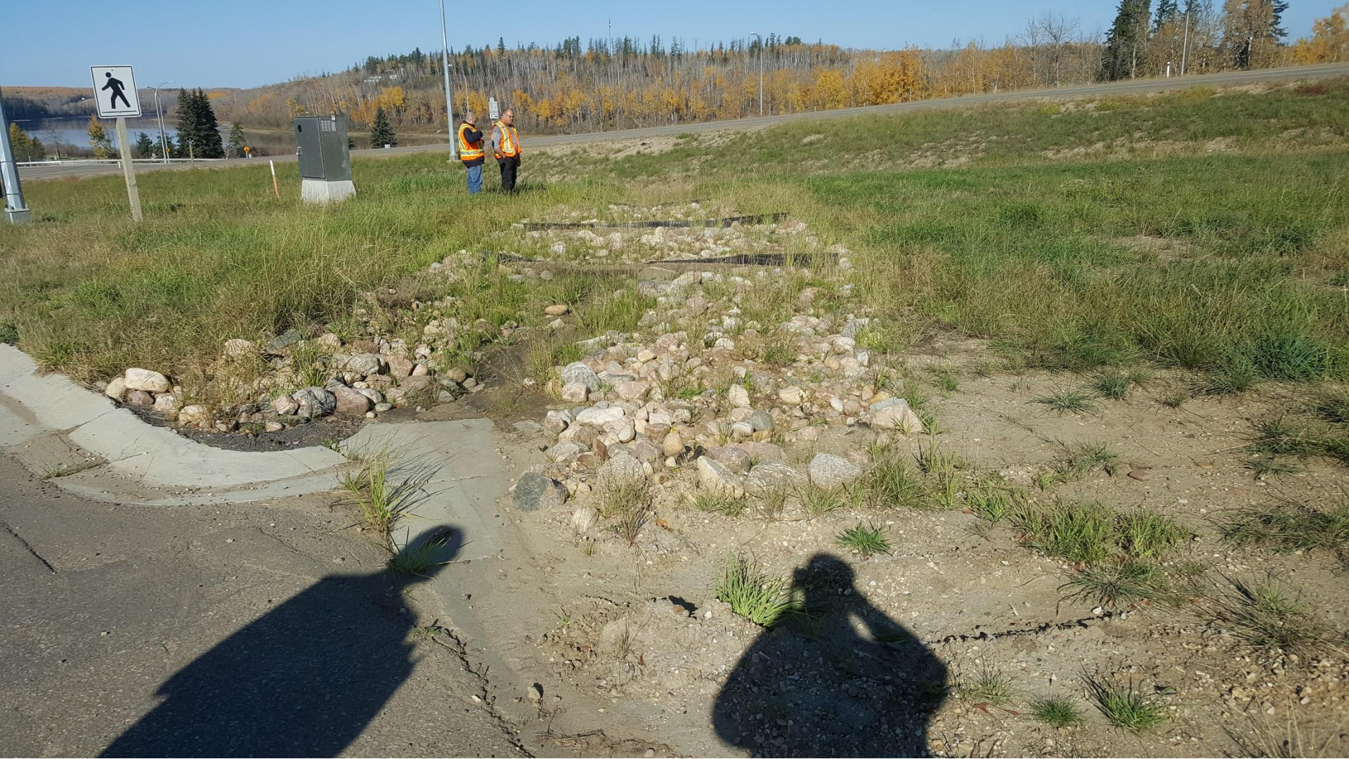
50 Avenue: sediment accumulation in channel added after runoff flooded electrical box
