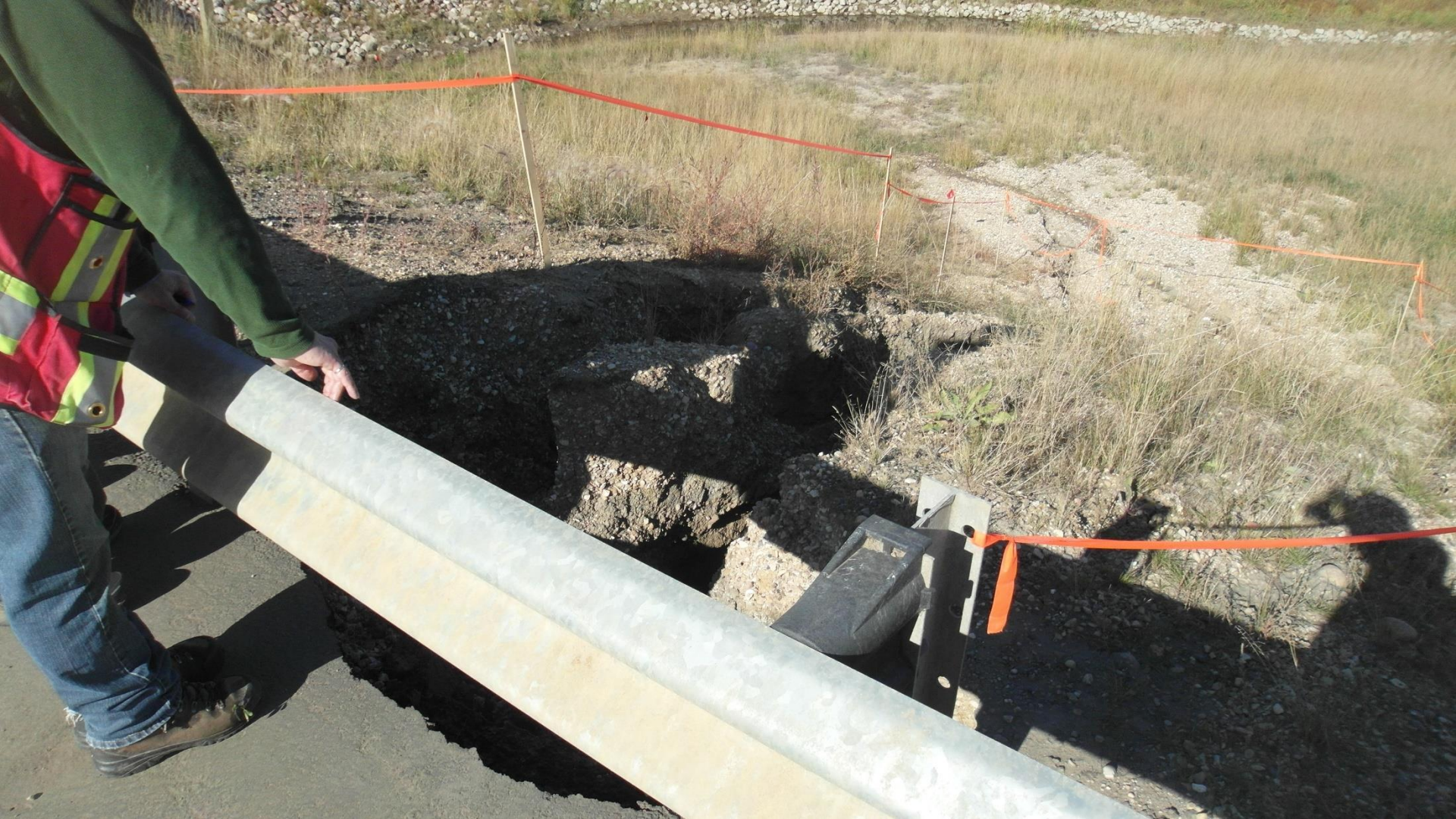
Hwy 55 NE corner of bridge: erosion encroaching
