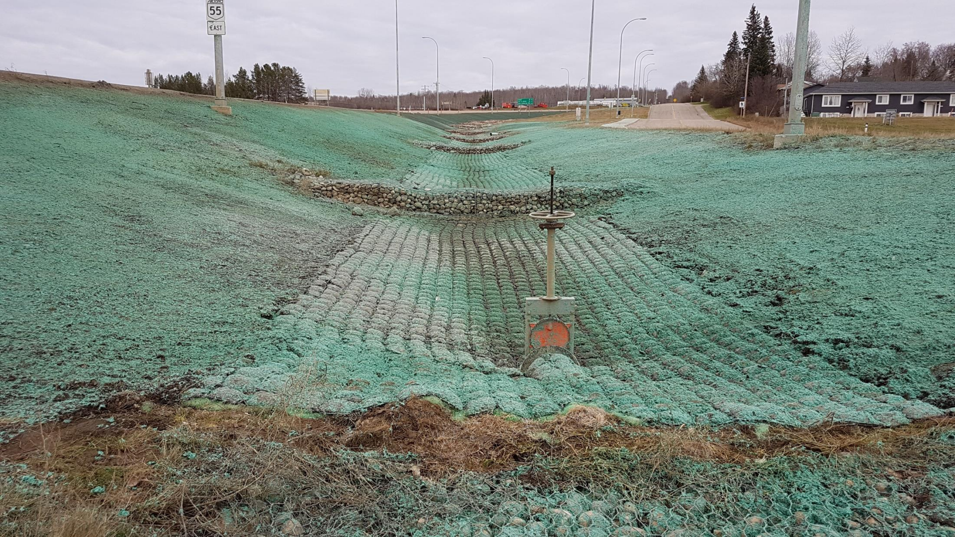
Hwy 55 south ditch: Flexamat and hydroseed
