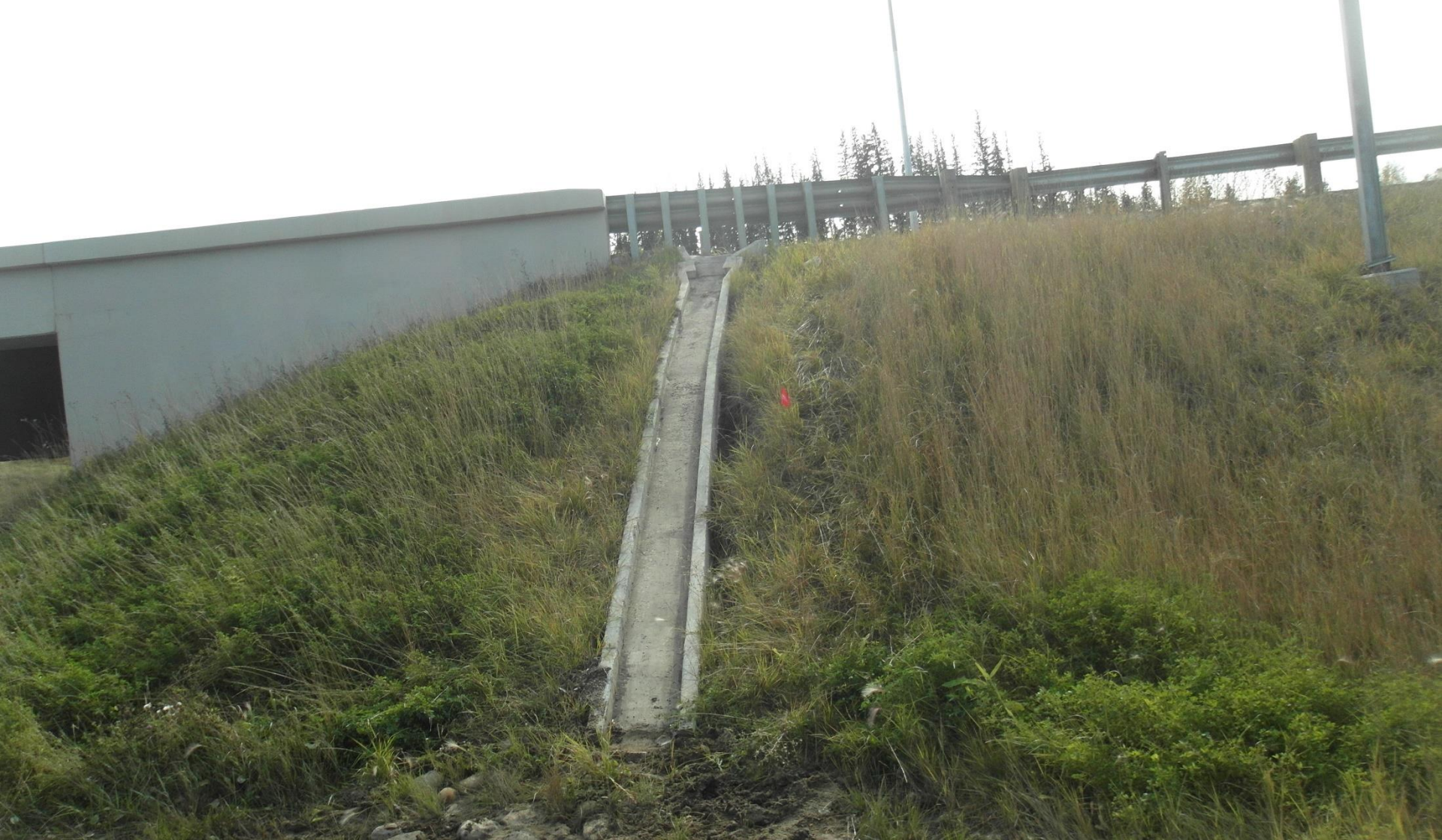
Hwy 55 NW corner of bridge – undercutting trough
