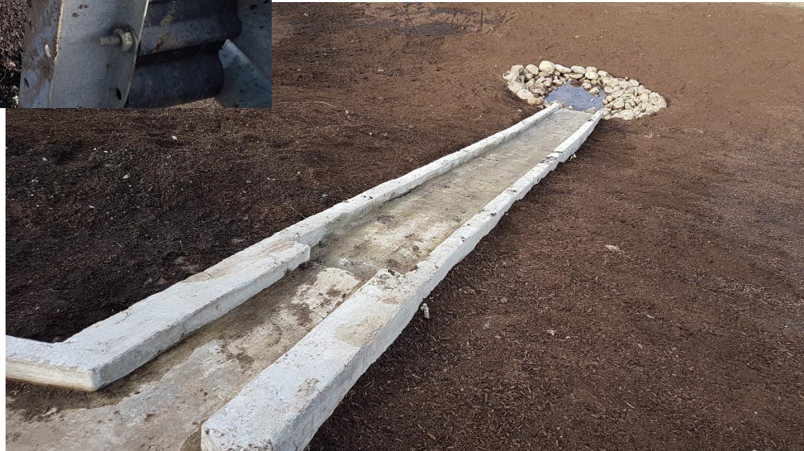
NE corner – new drain trough with dissipation bowl
