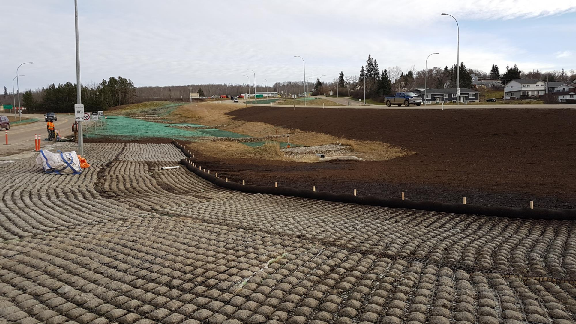
Hwy 813: Flexamat, compost sock, compost blanket, and hydroseed
