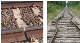
Figure 1: Abnormal stresses in the rail steel can result in rail break (left) and buckled tracks (right)
