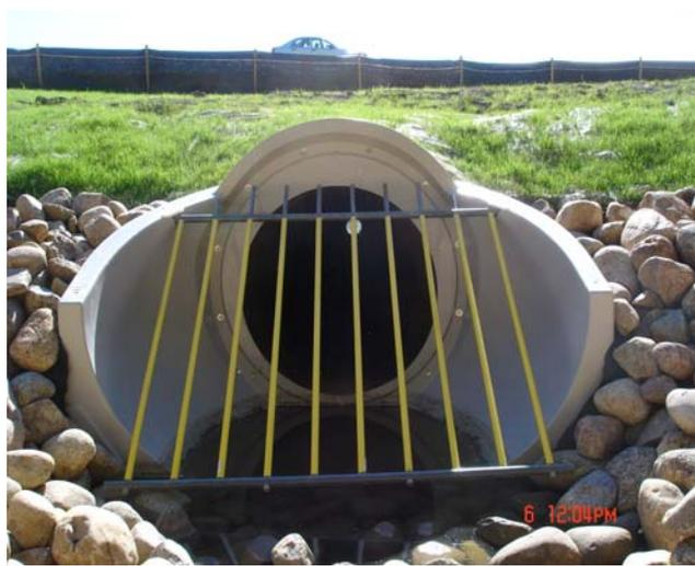
Upstream end, End treatment with grate (1200 mm dia.)
