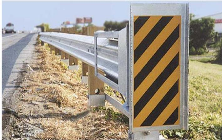
The Extruder Terminal (ET-Plus) is a proprietary, energy-absorbing, gating, tangent end treatment.
