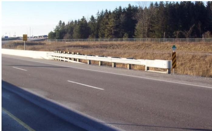
The Crash Cushion Attenuating Terminal (CAT-350) is a proprietary, energy-absorbing, gating, redirective terminal designed to shield narrow hazards.
