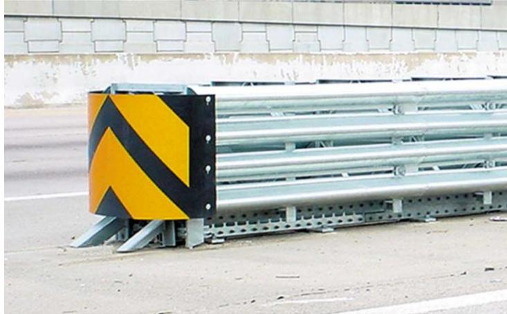
The Trinity Attenuating Crash Cushion (TRACC) is a proprietary, energy-absorbing, restorable, non-gating, redirective end treatment designed to shield narrow hazards.
