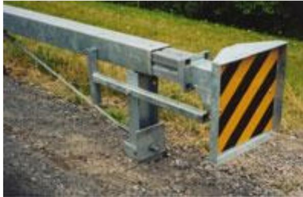
The Bursting Energy Absorbing Terminal (BEAT) system is a proprietary, energy-absorbing redirective terminal designed to shield the end of the Box Beam Barrier.
