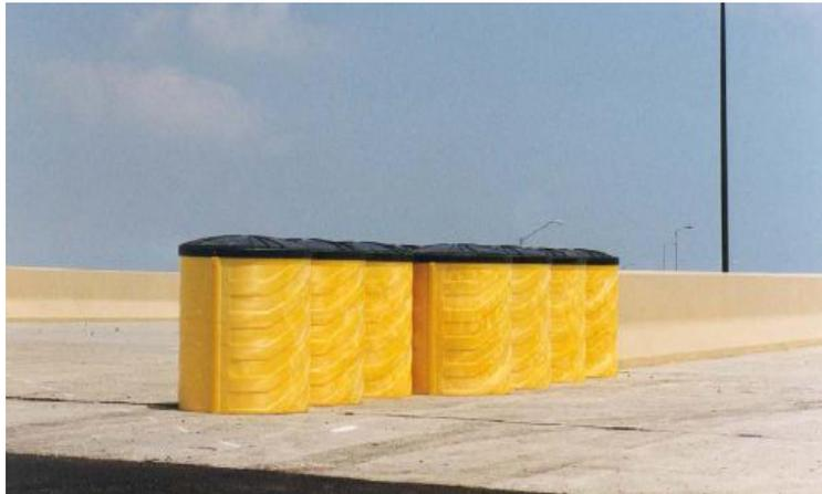
Sand Barrel Systems refer to a family of proprietary, non-redirective, and gating, end treatments.
