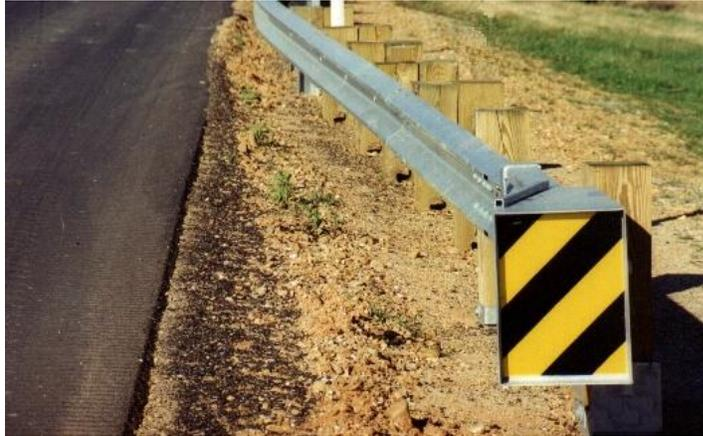
The Flared Energy Absorbing Terminal (FLEAT) is a proprietary, energy-absorbing, gating, flared end treatment.
