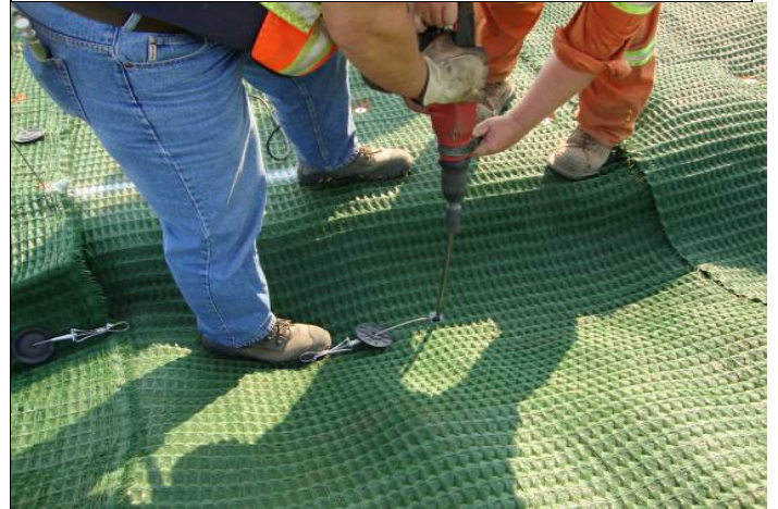
Hilti hammering the duckbill anchors
