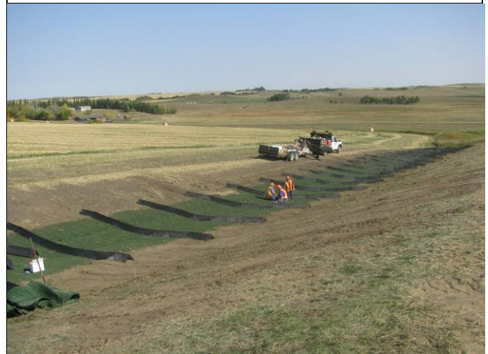
Placement of anchor pins
