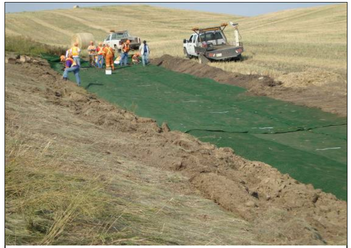
H614:02 – 2009 During construction
