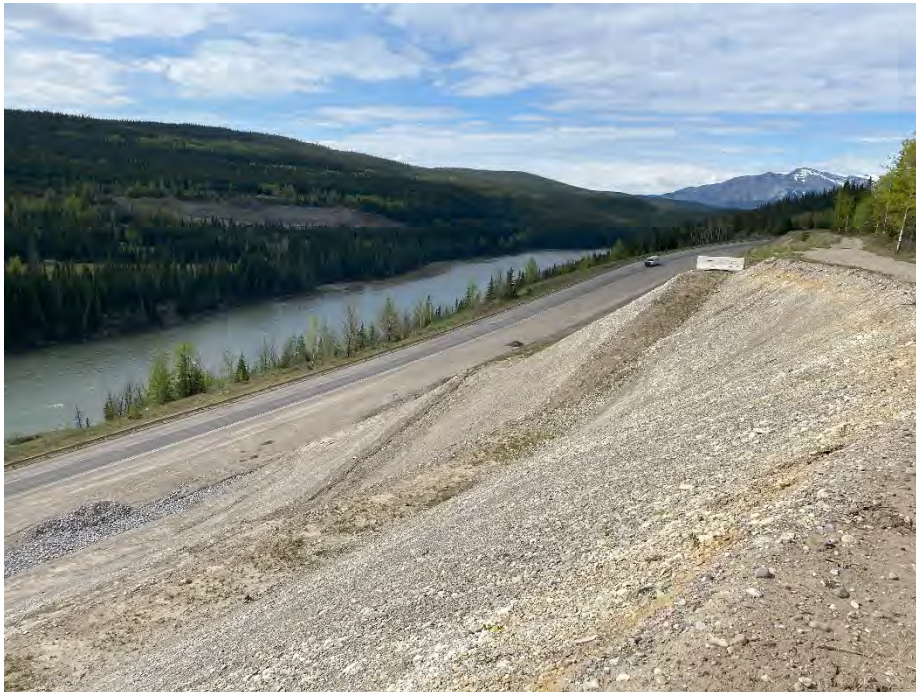
Photo 14: Highway and backslope, looking southwest from crest of backslope.
