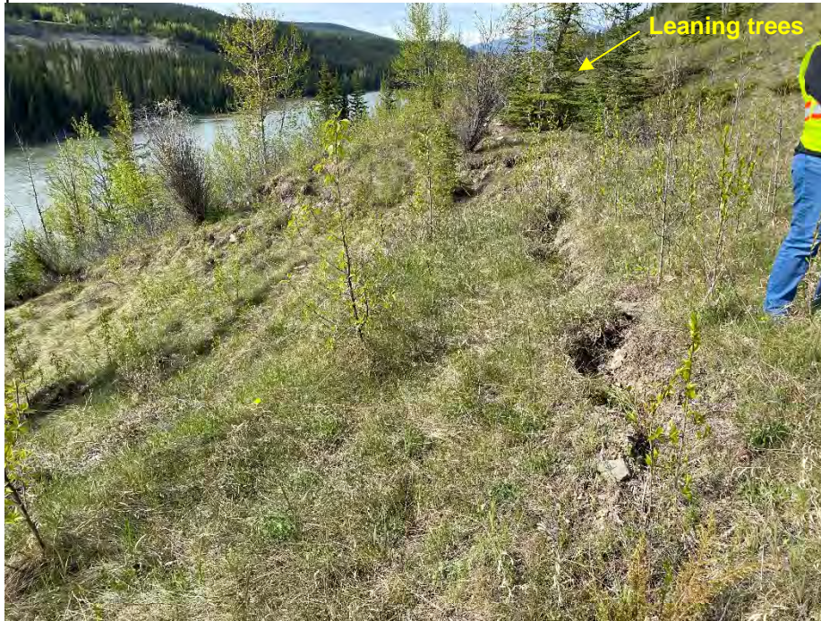
Photo 5: Ground crack at ridge location near the centre of the east landslide. Leaning trees in background. Looking southwest.
