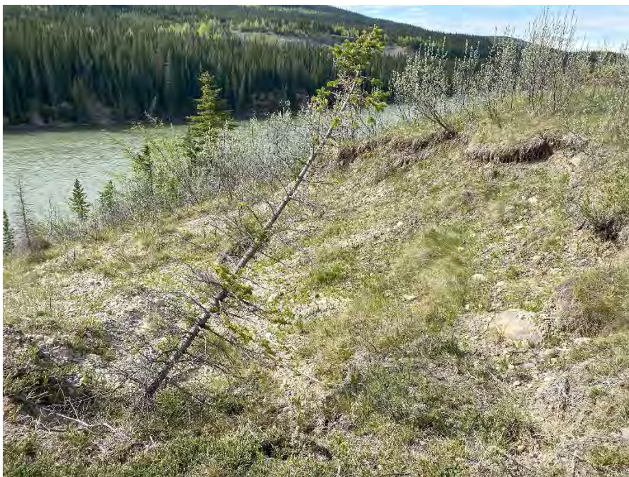
Photo 8: Scarp at far east extent of eastern slide zone. Looking south.
