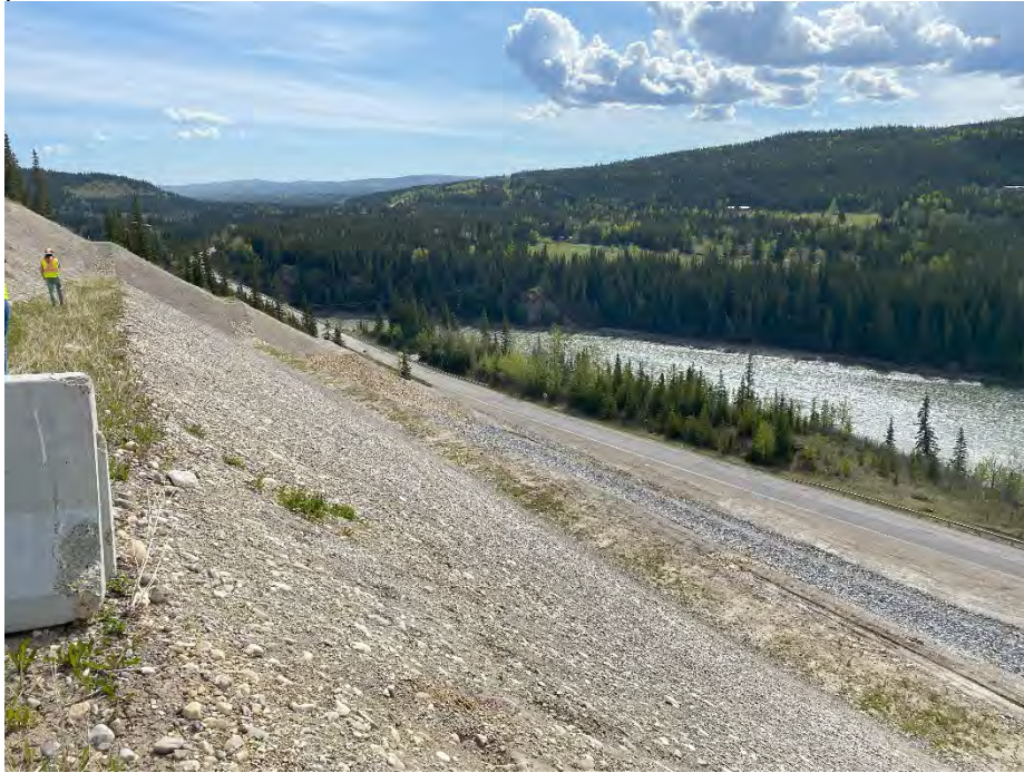
Photo 15: Highway and backslope, looking east from crest of backslope.
