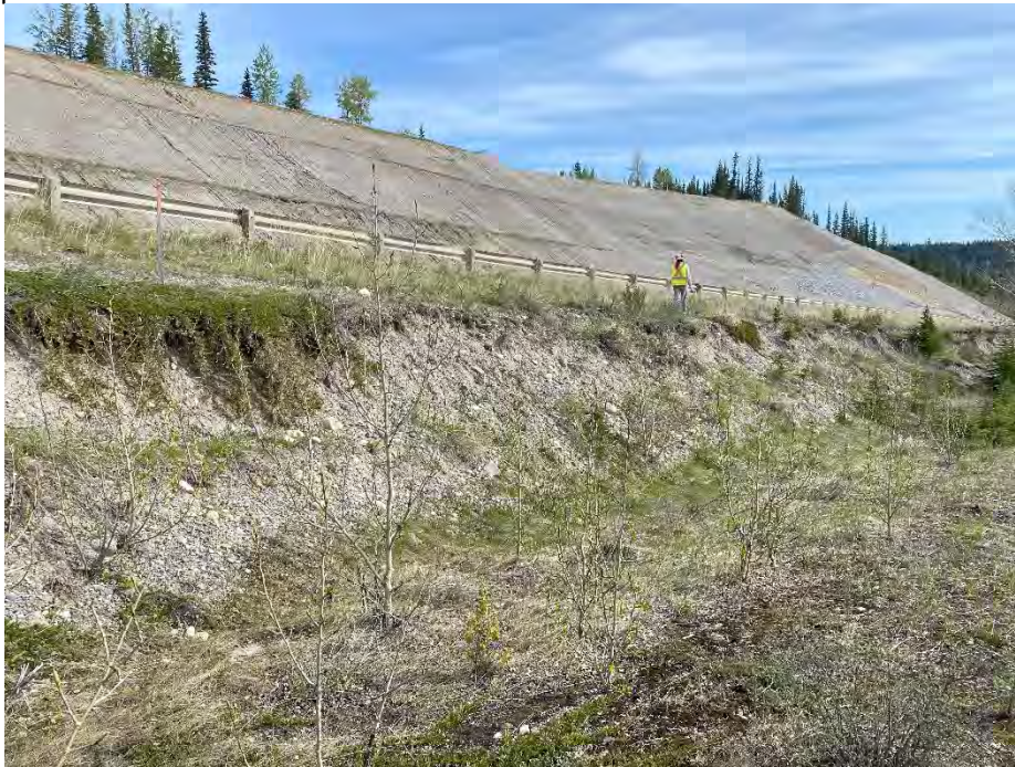
Photo 7: Scarp along highway, near guardrail. Looking northeast.
